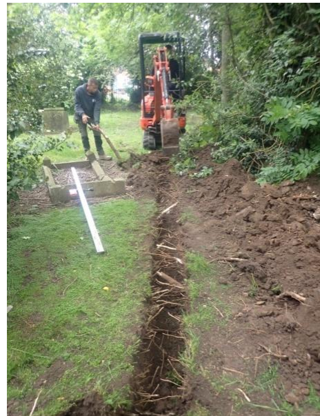
Plate 15: Excavation of the service trench, from the west
