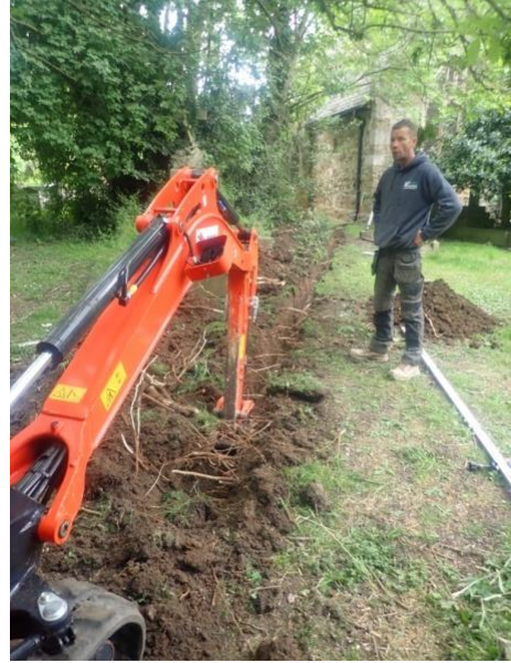
Plate 30: Excavation of the service trench, from the east
