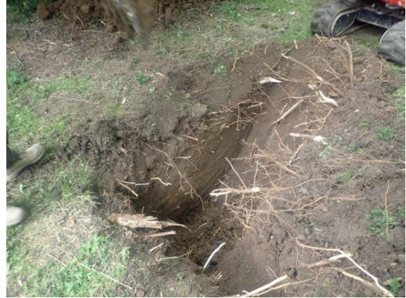
Plate 35: Excavation of the soakaway , from the north
