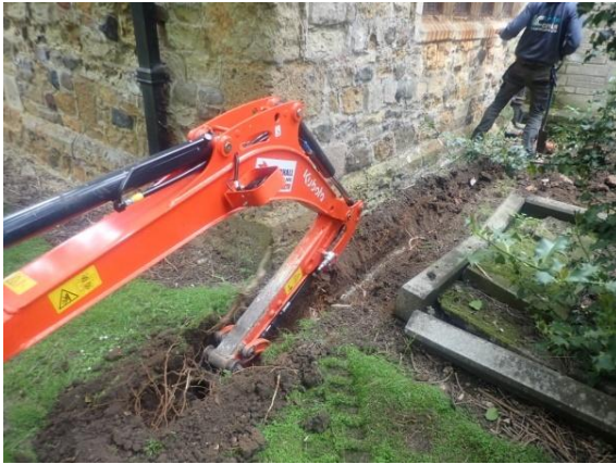
Plate 8: Excavation of the service trench, from the south-east
