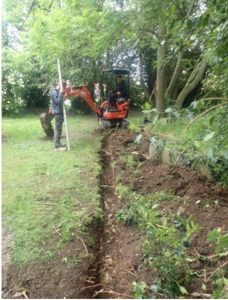
Plate 24: Excavation of the service trench, from the west
