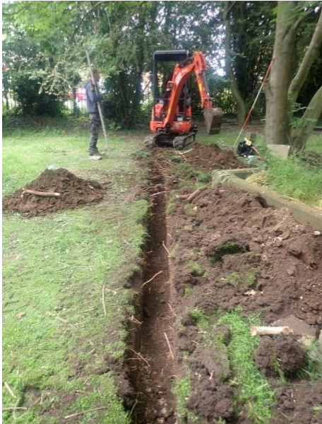
Plate 29: Excavation of the service trench, from the west
