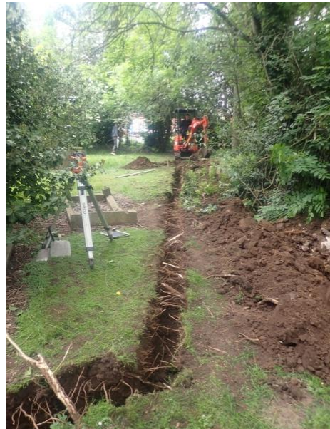
Plate 27: Excavation of the service trench, from the west
