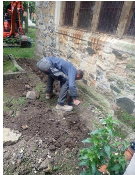
Plate 6: Excavation of the service trench, from the north-east
