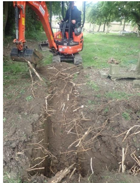
Plate 36: Excavation of the soakaway , from the north
