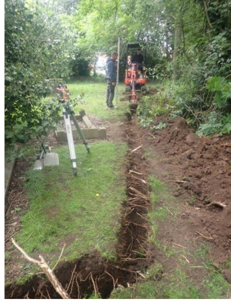
Plate 22: Excavation of the service trench, from the west
