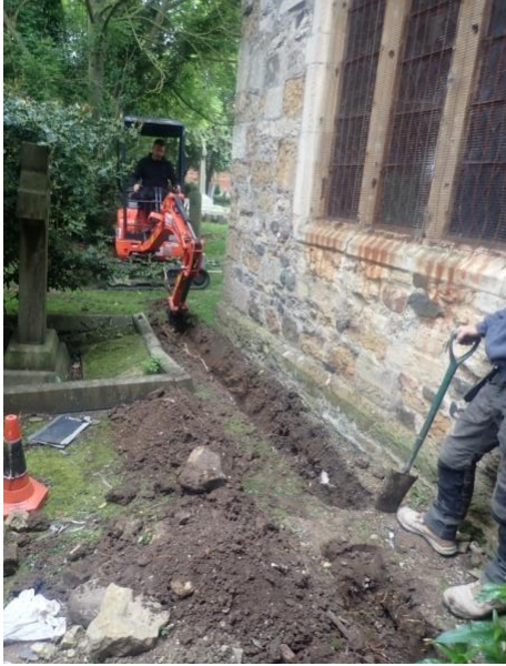
Plate 7: Excavation of the service trench, from the north-east
