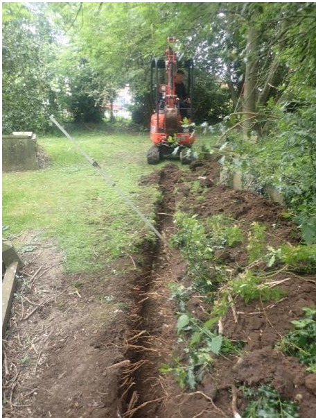
Plate 21: Excavation of the service trench, from the west
