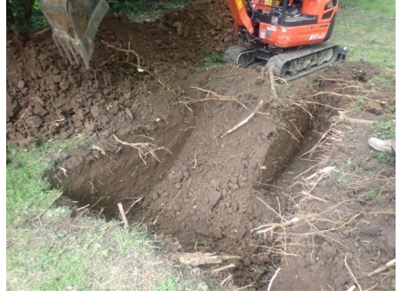
Plate 39: Excavation of the soakaway, from the north
