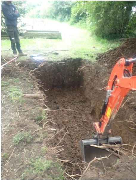
Plate 43: Excavated soakaway, from the south
