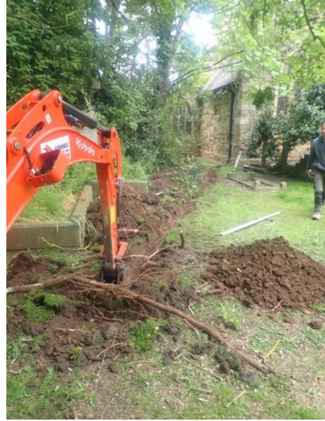
Plate 26: Excavation of the service trench, from the east
