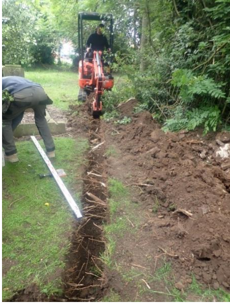
Plate 16: Excavation of the service trench, from the west
