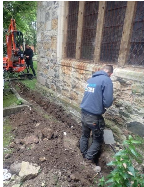
Plate 10: Excavation of the service trench, from the north-east
