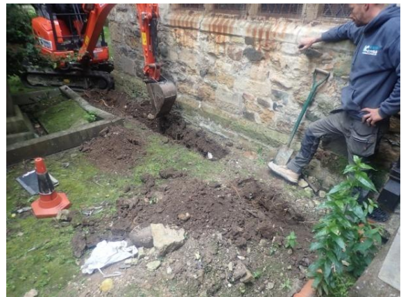
Plate 5: Excavation of the service trench, from the north-east
