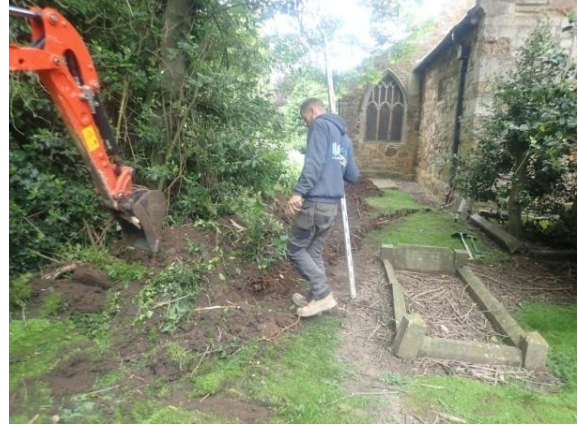
Plate 18: Excavation of the service trench, from the east
