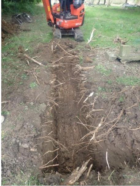
Plate 37: Excavation of the soakaway, from the north
