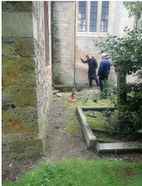
Plate 2: Pre-groundworks, from the south
