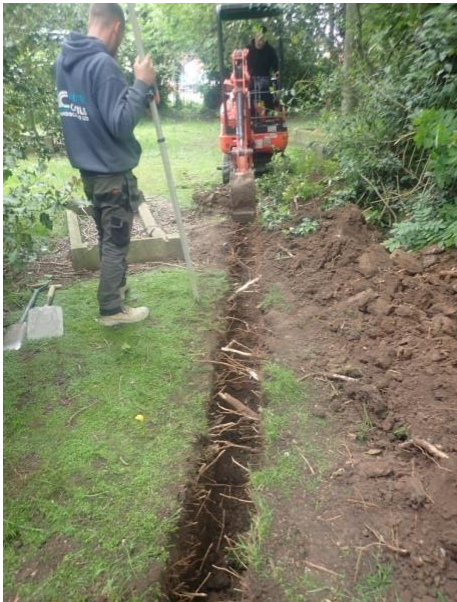
Plate 17: Excavation of the service trench, from the west
