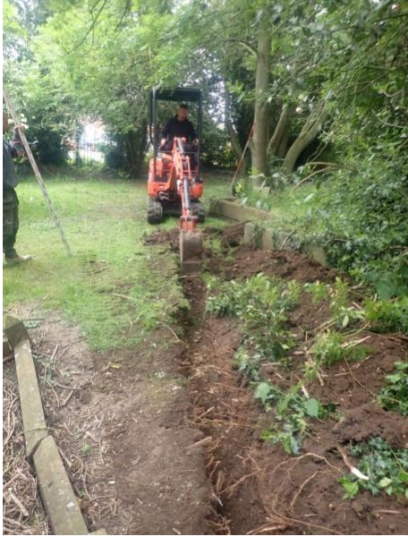
Plate 20: Excavation of the service trench, from the west
