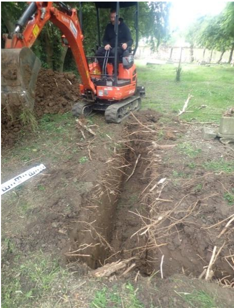
Plate 38: Excavation of the soakaway, from the north
