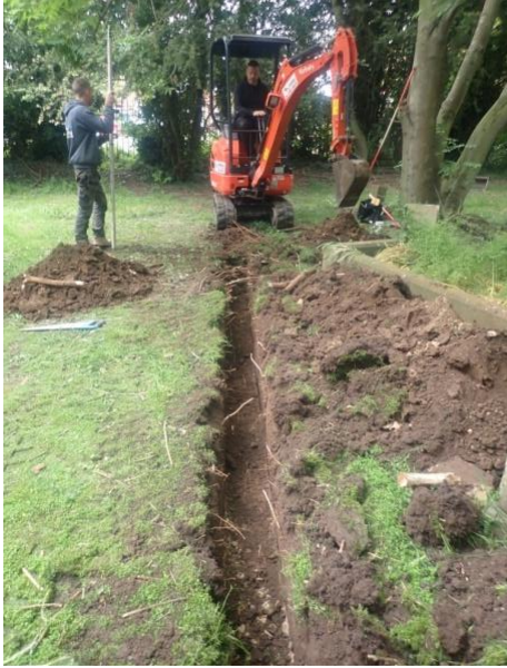
Plate 28: Excavation of the service trench, from the west
