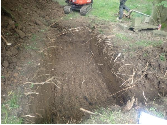
Plate 42: Excavated soakaway, from the north
