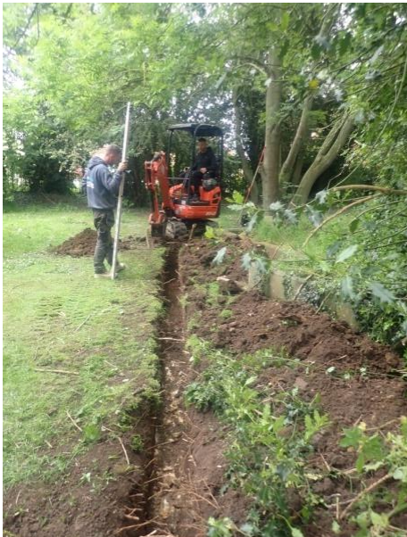
Plate 25: Excavation of the service trench, from the west
