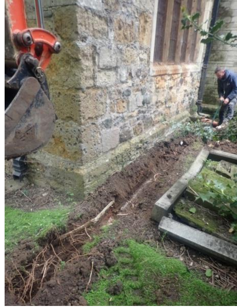
Plate 9: Excavation of the service trench, from the south-east
