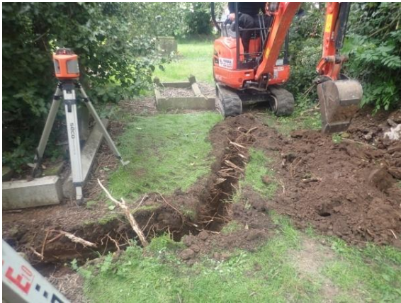
Plate 12: Excavation of the service trench, from the west
