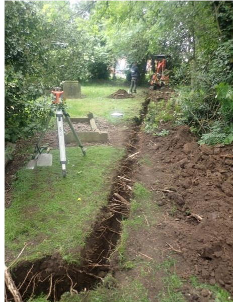
Plate 31: Excavation of the service trench, from the west
