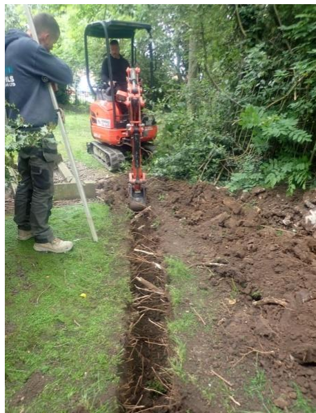
Plate 13: Excavation of the service trench, from the west
