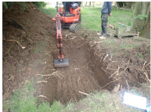
Plate 41: Excavation of the soakaway, from the north
