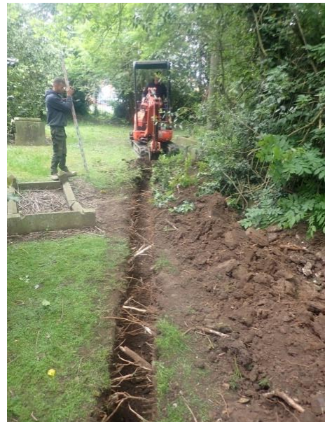
Plate 19: Excavation of the service trench, from the west
