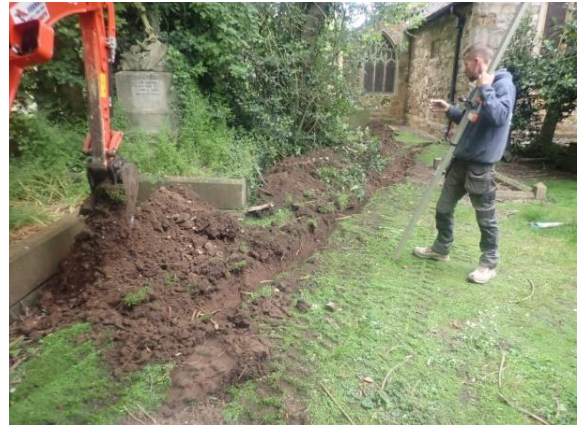
Plate 23: Excavation of the service trench, from the east
