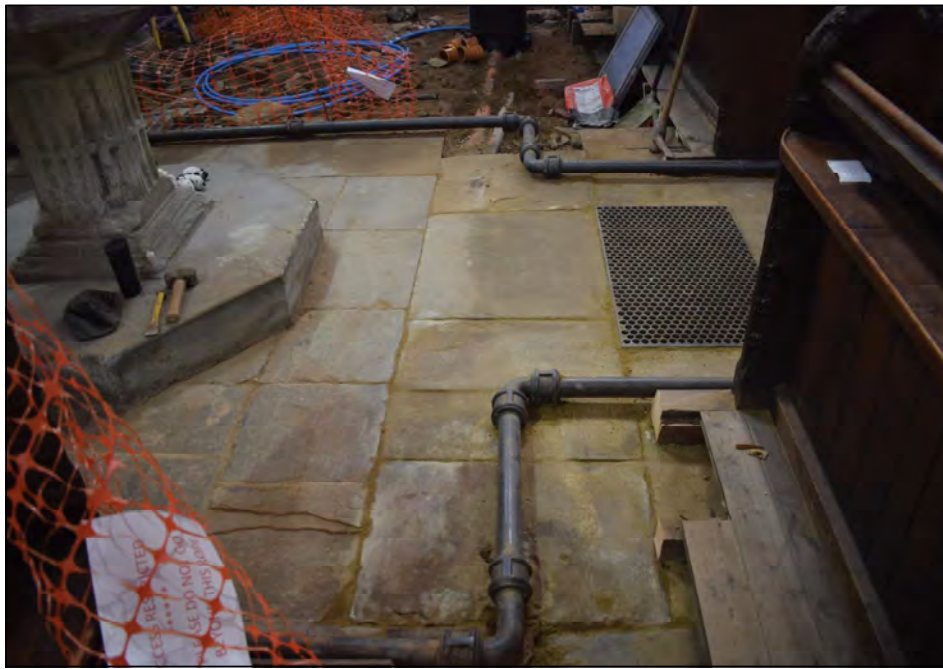
Plate 8. Flagstones replaced over Trench 4, looking north
