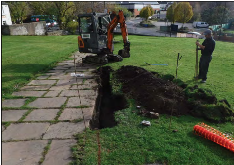
Plate 2. Trench 2 being excavated, looking southeast
