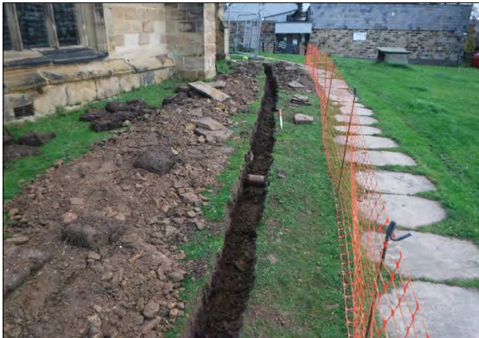
Plate 4. Trench 3 with modern drainage pipe in the base, looking northeast
