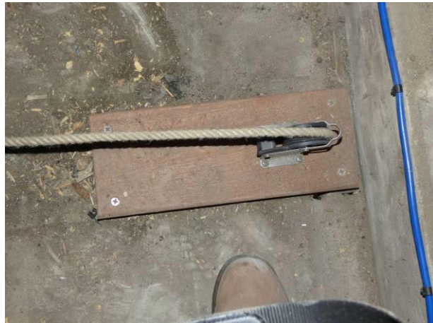
The old rope pulleys left in situ and the new pulleys for the lever safety clappers mounted on the floor. These pulleys are from the Bartol range design for marine usage.
