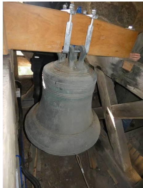
The new "dead stocks" of sapele fitted after the bells had been drilled for centre holes and the cast in staples removed as much as possible. Also the new galvanized supporting ironwork.
