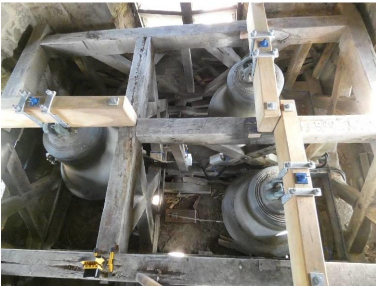
The new "dead stocks" of sapele fitted after the bells had been drilled for centre holes and the cast in staples removed as much as possible. Also the new galvanized supporting ironwork.
