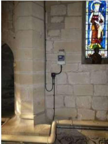
The control unit mounted on the West wall adjacent to the tower doorway and a close up of the Apollo III control unit. These units now have touch screen operation.
