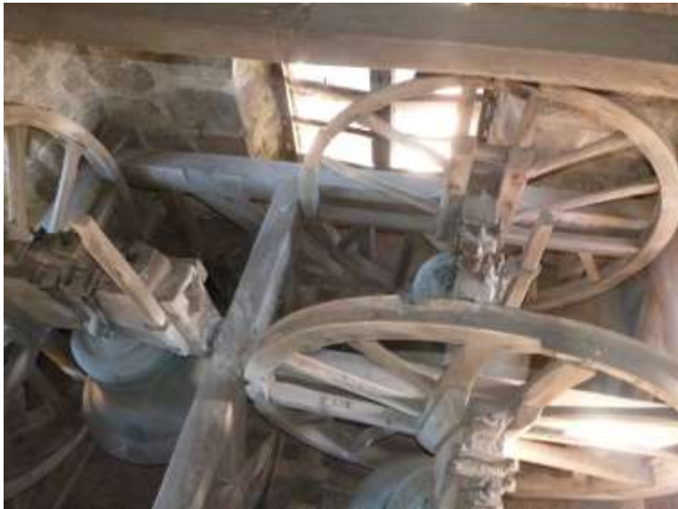
The bells with their derelict fittings and rot at the end of the headstocks
