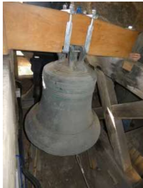
The new “dead stocks” of sepele fitted after the bells had been drilled for centre holes and the cast in staples removed as much as possible. Also the new galvanised supporting ironwork.
