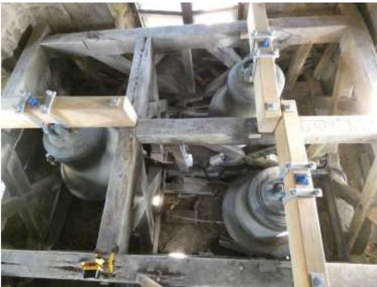
The new “dead stocks” of sepele fitted after the bells had been drilled for centre holes and the cast in staples removed as much as possible. Also the new galvanised supporting ironwork.
