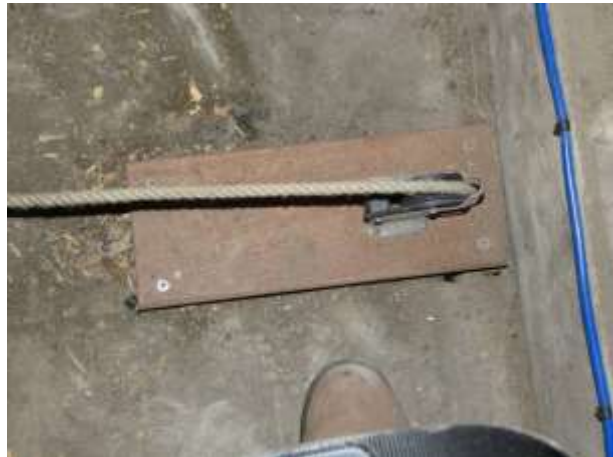
The old rope pulleys left in situ and the new pulleys for the lever safety clappers mounted on the floor. These pulleys are from the Bartol range designed for marine usage.
