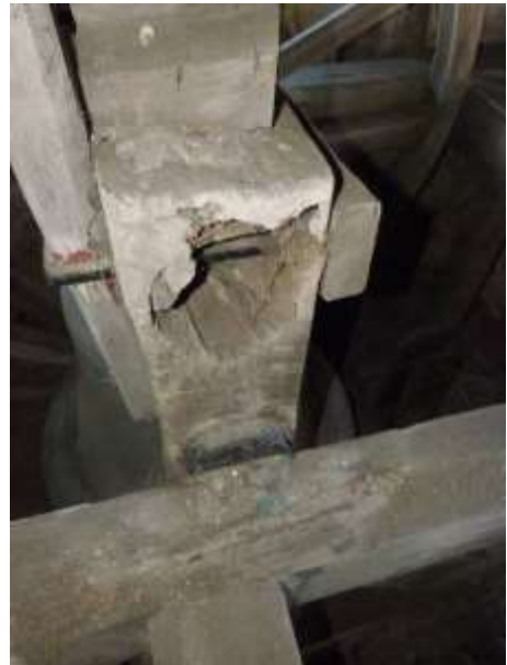
The bells with their derelict fittings and rot at the end of the headstocks
