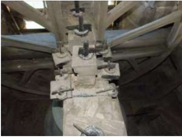
Wedge bolts and old blacksmiths strap bolts. (Only the visible parts had been painted!)
