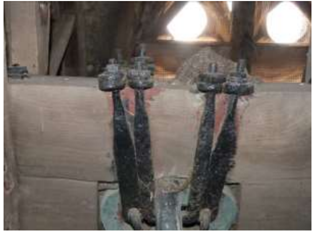
Wedge bolts and old blacksmiths strap bolts. (Only the visible parts had been painted!)
