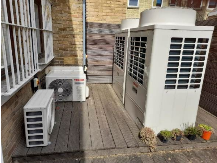
Examples of external units for AASHP comprising of three smaller 3kW units (delivering 10kW each) and two larger 10kW units (37.5kW output each).
