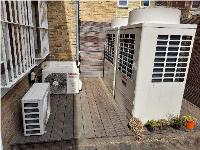
Examples of external units for AASHP comprising of three smaller 3kW units (with 10kw output each) and two larger 10kW units of 37.5kW output each.
