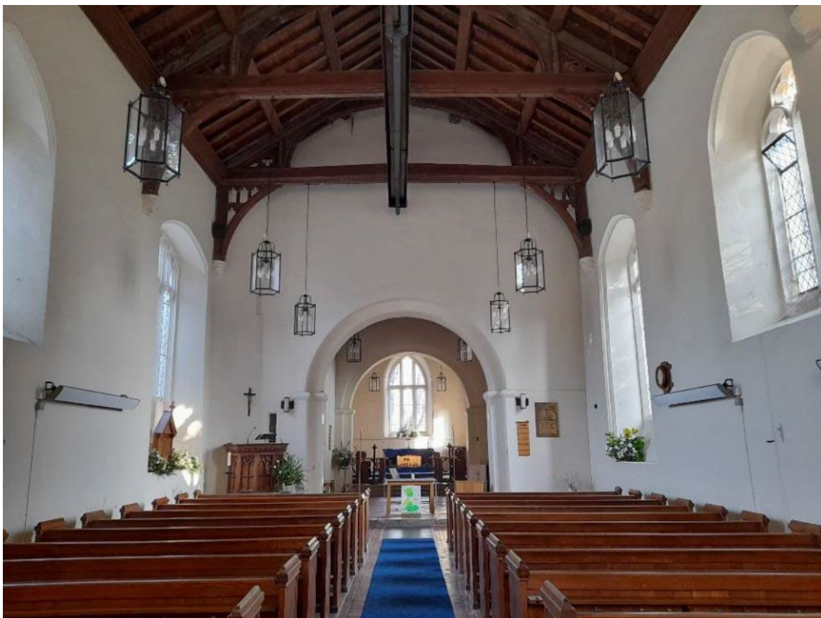
Above, looking east. The nave is heated by wall mounted radiant heaters.
