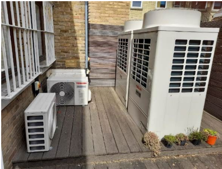
Examples of external units for AASHP comprising of three smaller 3kW units of 10kW output and two larger 10kW units of 37.5kW output
