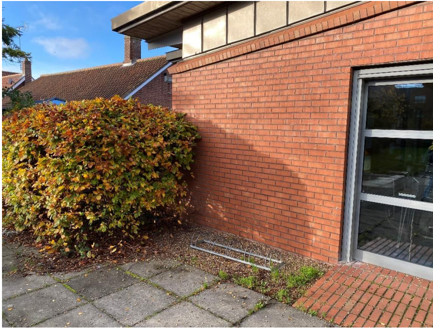
Area external to church for consideration for battery storage unit
