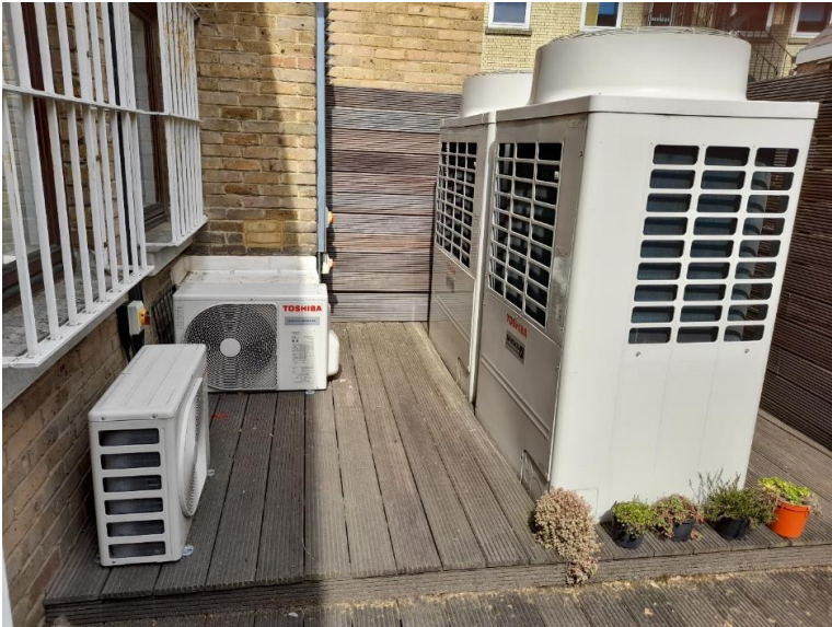
Examples of external units for AWSHP comprising of three smaller 3kW units and two larger 10kW units.
