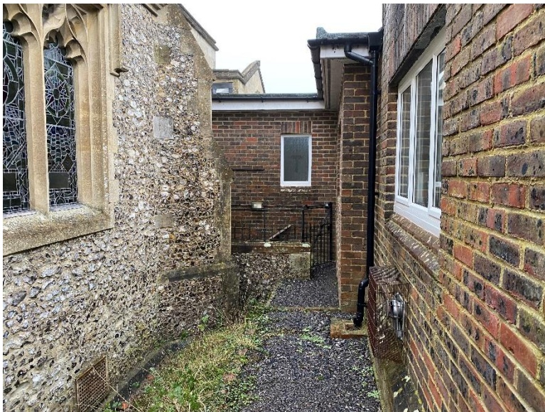
Area identified where external units could be placed with minimal intrusion.
