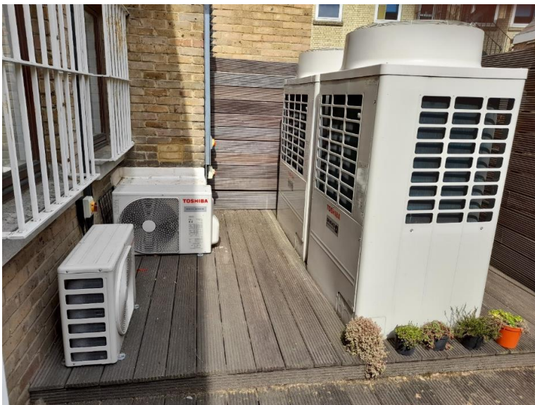
Examples of external units for AASHP comprising of three smaller 3kW units and two larger 10kW units.
