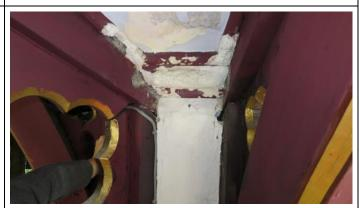
Photo 085 shows the external detail above obs 12 and 13 which is prone to blockage and was holding some detritus and standing water at the time of survey.
