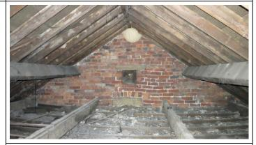
The common ceiling joists have bowed away from the beam. It seems as if the nails through the common rafters have pulled out of the underside of the ceiling beam. Consequently, the ceiling cannot take any amount of weight.
