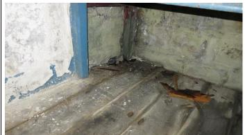
Photos 046 shows the underside of the floor at this point. It is likely at least 2 or 3 common joist bearings are decayed in the S wall and the principle floor beam (arrowed opposite) has lost most of its sapwood to wet rot decay within the wall and will therefore require additional support.
