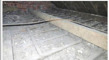
Photo 042 looking into the N transept. Again the ceiling structure seems to have pulled away from the ceiling beam and again no access was attempted. The purlin and ceiling beam bearings appear sound.
