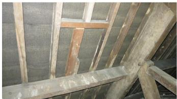
Photo 048 shows the purlin bearing adjacent to an area of water penetration (ob 17 below). The softwood purlin bearing has lost its outer (probably sapwood) edges within the wall.
