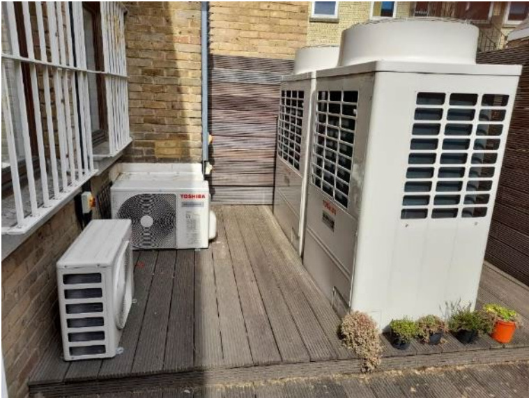
Examples of external units for AASHP comprising of three smaller 3kW units (of 10kW output each) and two larger 10kW units. (of 37kW output)
