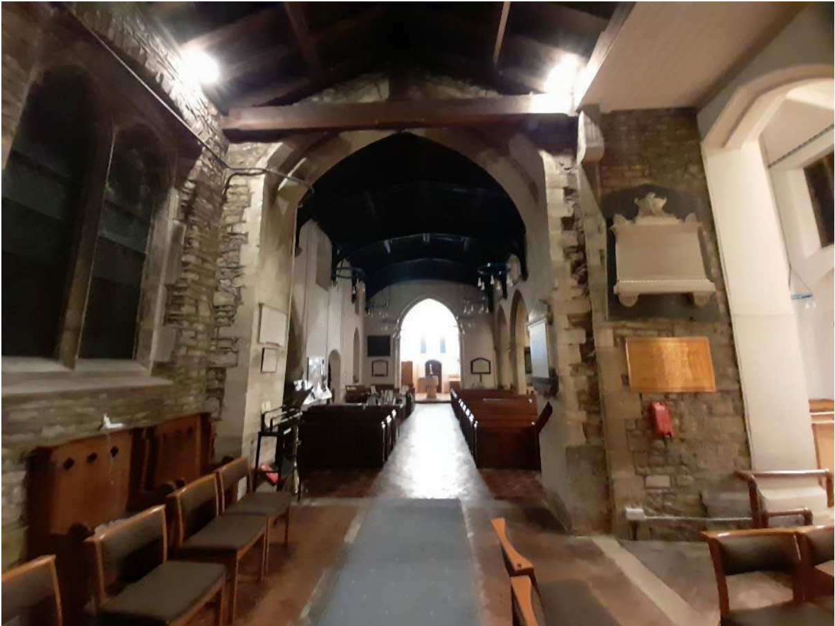
Above: Mediaeval portion of church looking west towards tower.
