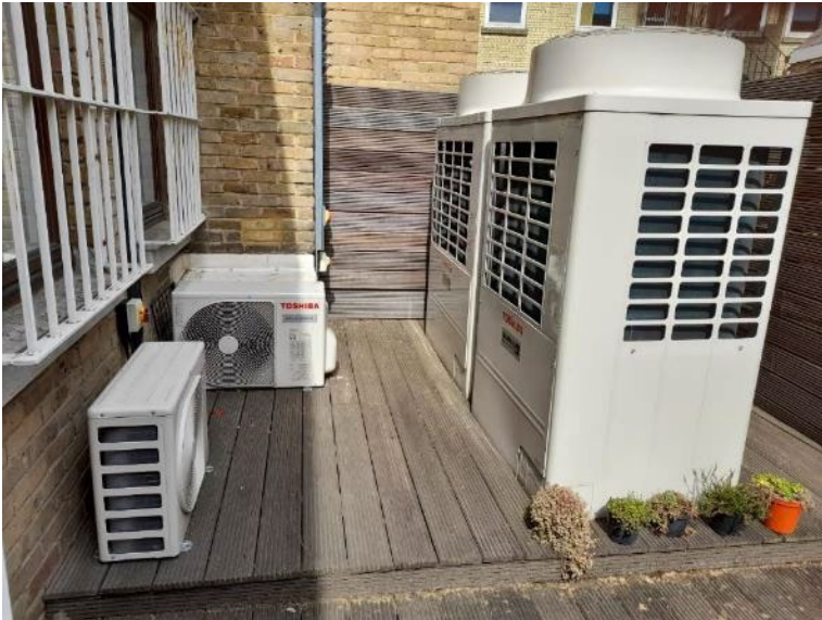
Examples of external units for AWSHP comprising of three smaller 3kW units and two larger 10kW units (which deliver 37kW output each).
