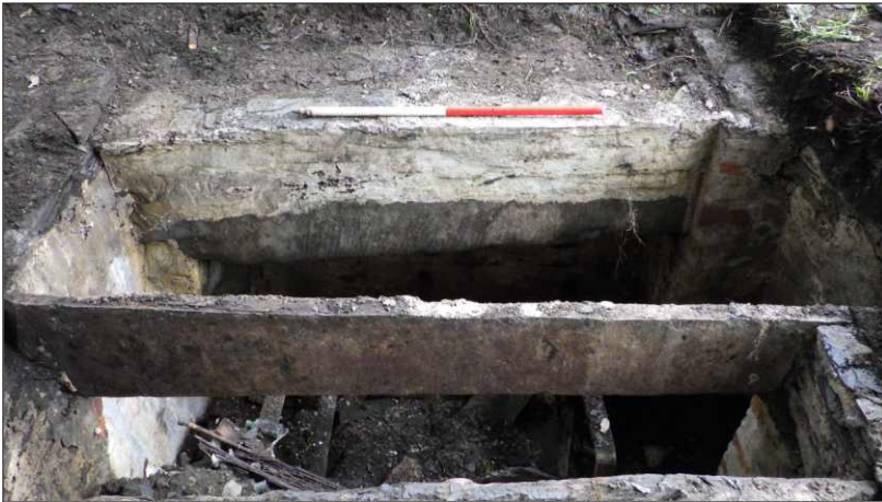
Plate 5: View of the burial vault with slate and concrete capping removed, looking southwest (1m scale)
