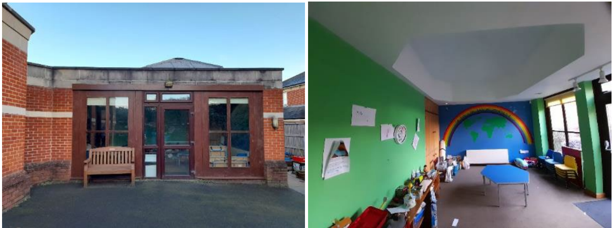
To the rear is a small room (the Playroom) which has potential for use for small meetings.
