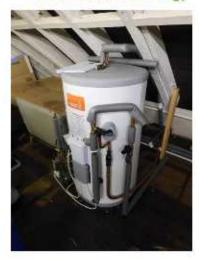
The current hot water strategy is that the hot water for the WC's and kitchen is heated from the gas boilers and stored in a small megaflow unit in the attic space.
