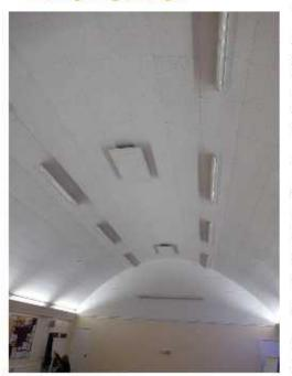
The lighting makes up a relatively large overall electricity load within the building. Good work has been done to convert the fittings in areas such as the lobby, trough uplights and some in the WC's to LED but the halls and kitchens are lit by relatively inefficient fluorescent fittings.
