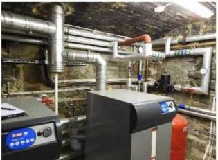
The church has a good gas boiler heating arrangement which was installed in April 2012 and consists of two Ideal iMax xtra F80 condensing boilers which serve radiators around the church. The church advises this provides adequate comfort and is only set to be on for when the church is occupied. This arrangement should be expected to last another 15 to 20 years.
