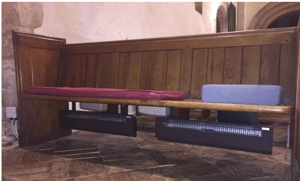
Brown BN Thermic 650W under pew heaters fixed to underside of pew seats for pews which have no solid backs.
