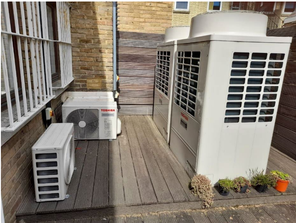
Examples of external units for ASHP comprising of three smaller 3kW units and two larger 10kW units.
