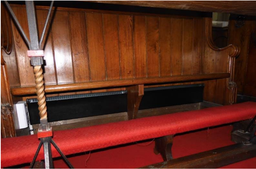
Black 650W Norel under pew heaters fitted to solid pew backs.
