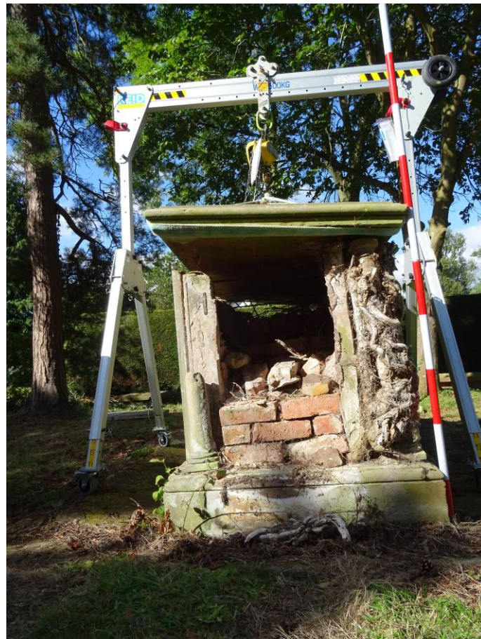
Plate 10. Dismantling of the tomb with the capstone suspended
