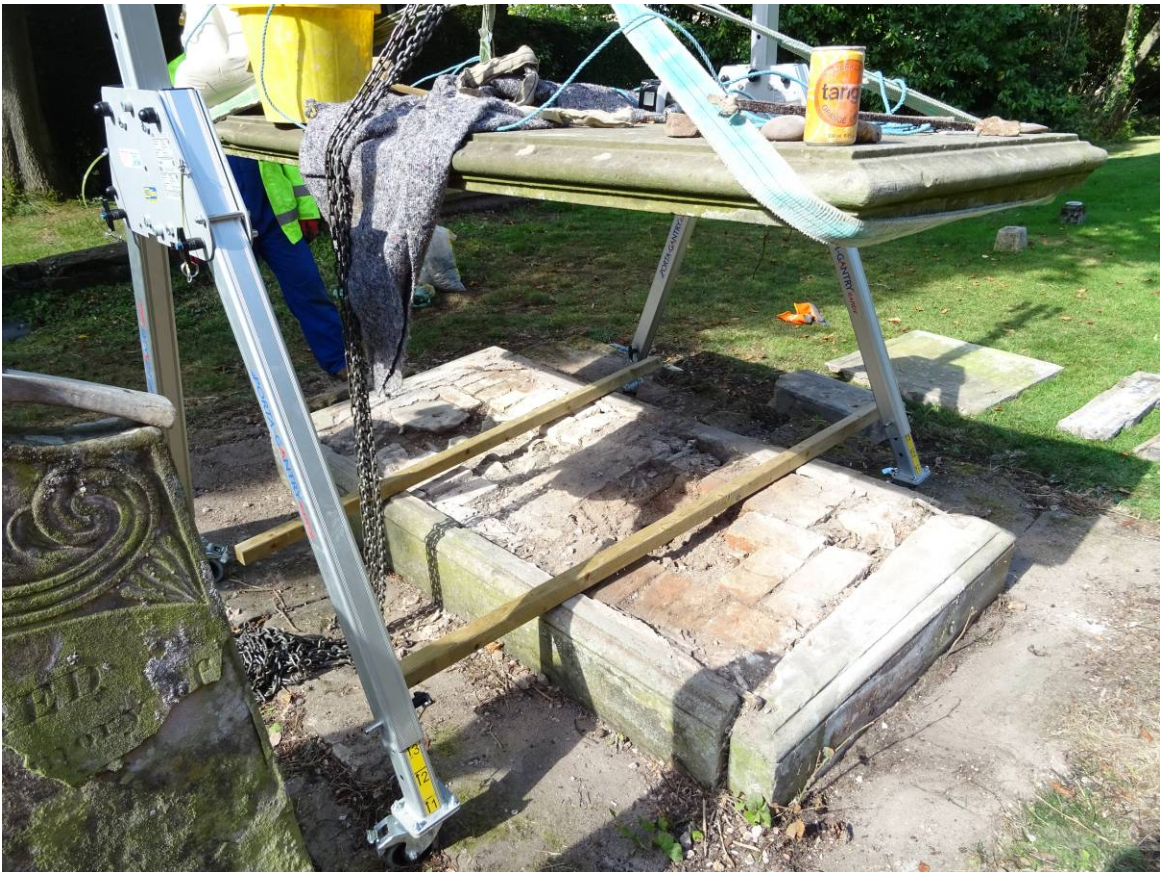
Plate 19. The complete removal of the various tomb sections, revealing the brick base
