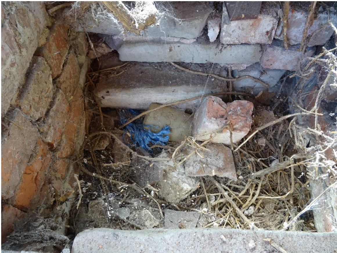
Plate 17. One of two rebuilt chambers within the core of the tomb
