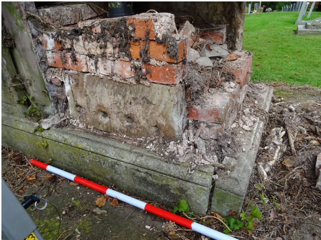
Plate 12. The inner core revealed, following the removal of the stone panels
