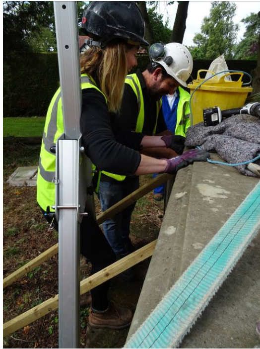
Plate 11. Steadying the capstone following the removal of the side panels
