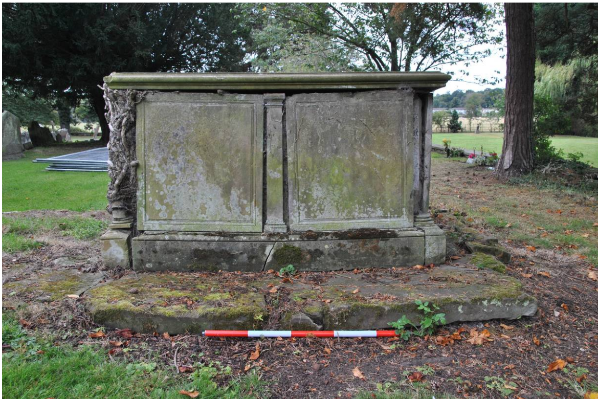
Plate 3. View of the northern side of the tomb before dismantling
