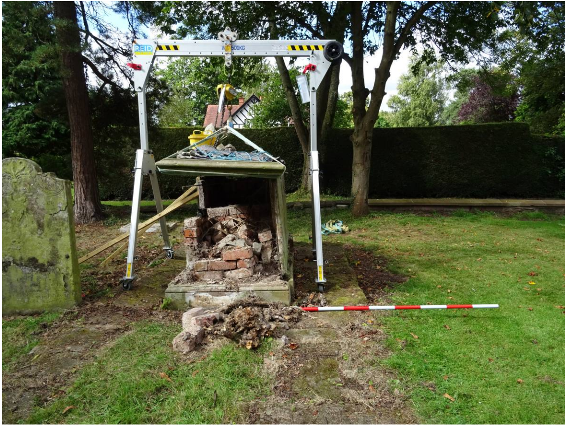
Plate 14. Dismantling of the tomb with several stone panels in place
