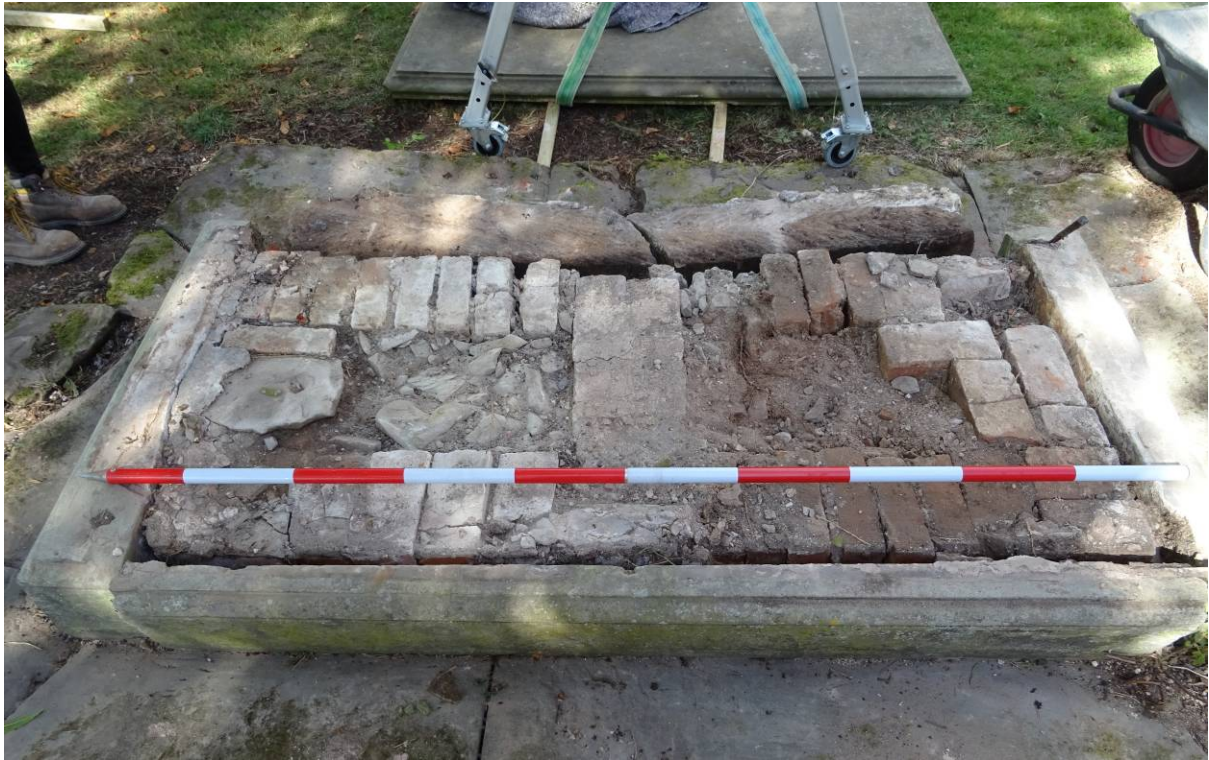
Plate 20. The base of the monument showing a re-set floor using building debris, enclosed by a moulded plinth
