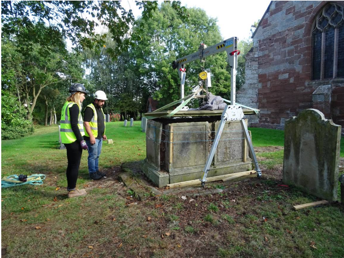
Plate 9. The lifting of the capstone and the steadying of the side panels
