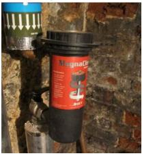
It is recommended that if the church chooses to retain the radiator network then a Magnetic Particle Filter is fitted to protect the system against further build up of magnetic sludge as has affected some of the radiators.
