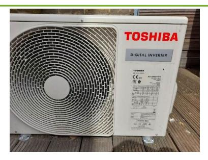
Three external units similar to the above, or one large unit would be needed to supply 30kW of heat.
