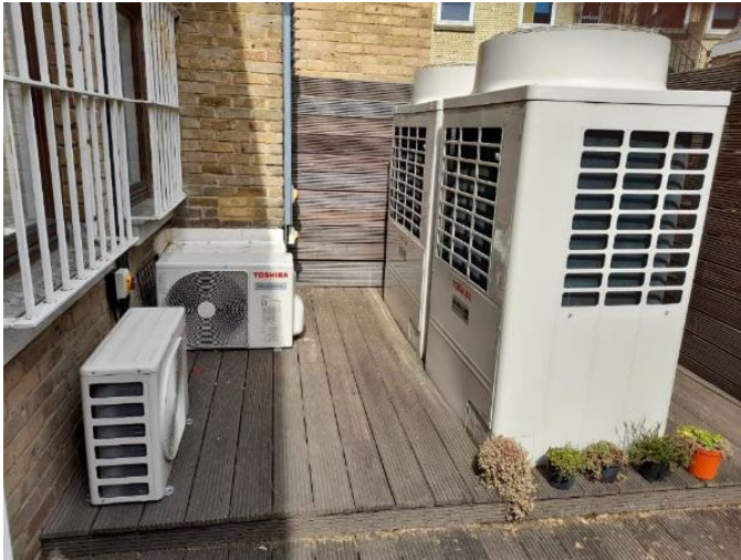
Examples of external units for ASHP comprising of three smaller 3kW units (10kW output each) and two larger 10kW units (37.5kW output each).
