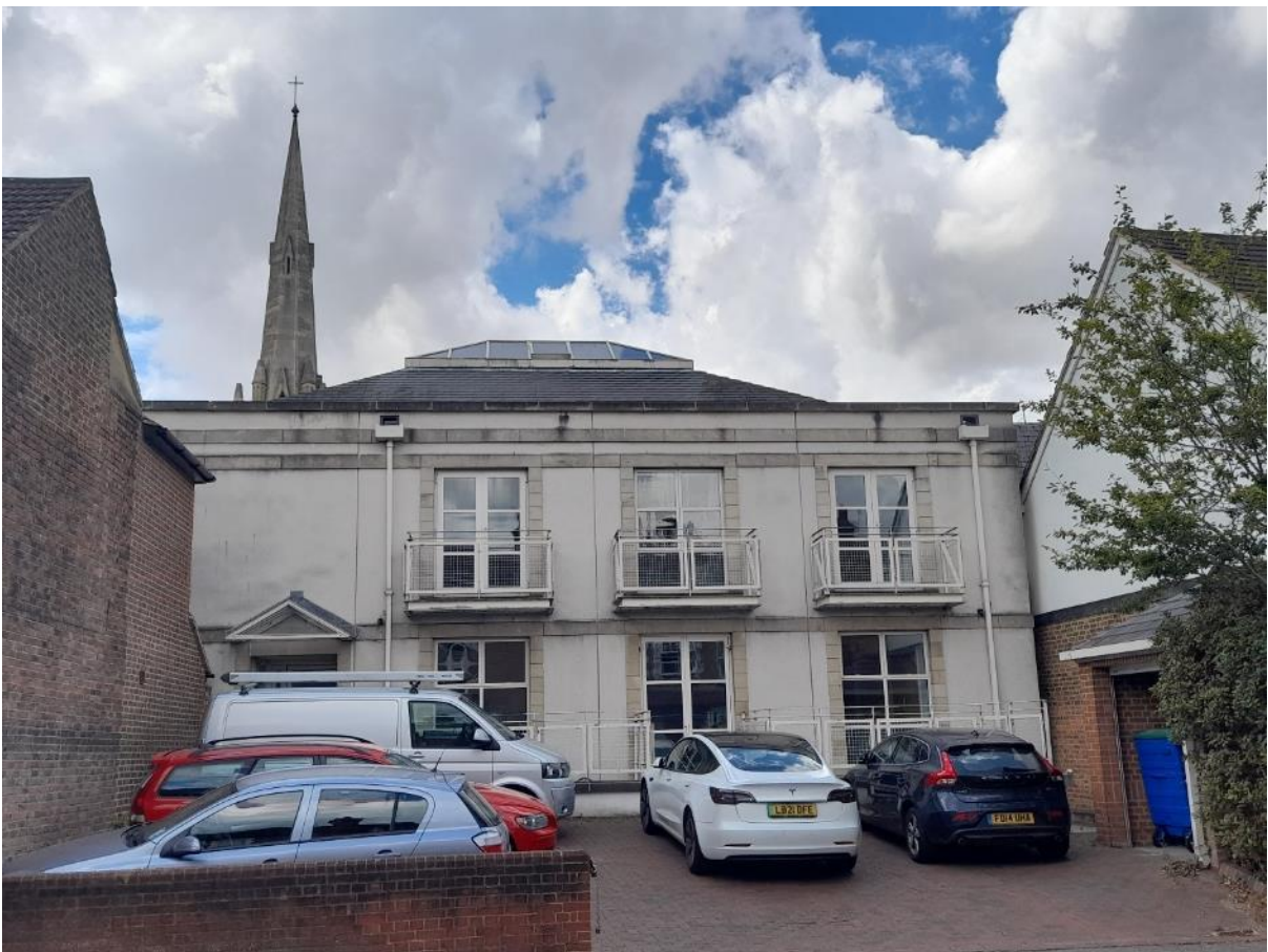
The rear of the hall is sunken one storey below the car park.
