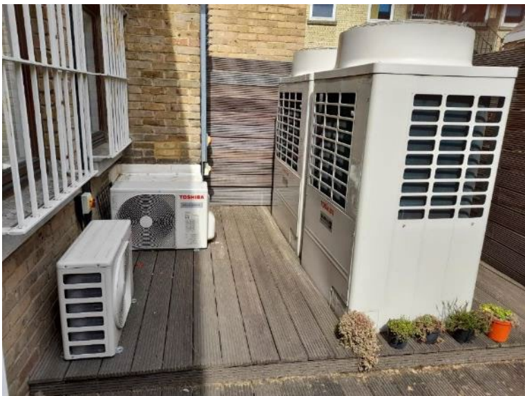
Examples of external units for ASHP comprising of three smaller 3kW units (with 10kW output each) and two larger 10kW units (with 37.5kW output each).
