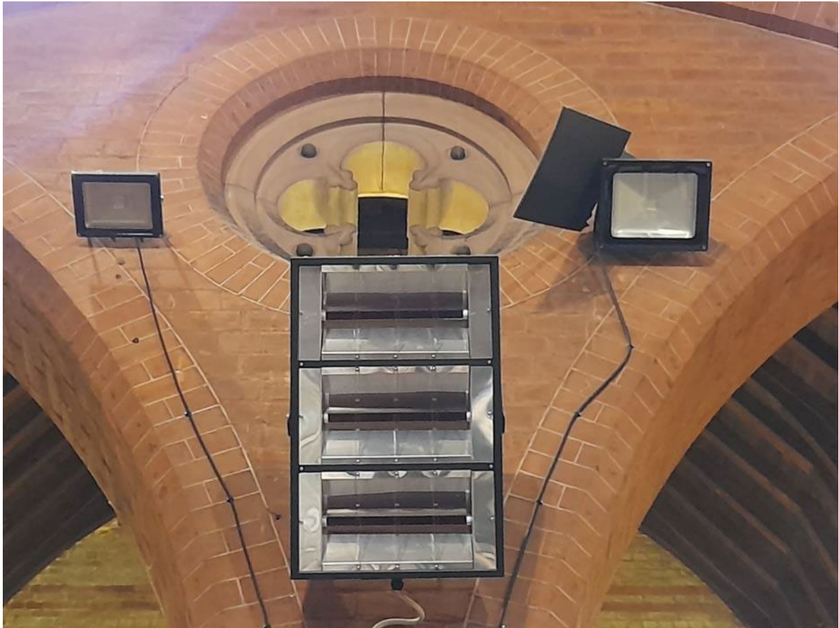
Above, triple quartz radiant heating unit.
