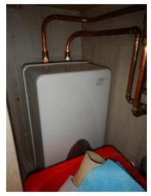
There are a number of electric point of use water heaters in the church hall to provide hot water for hand washing. This only needs to heat the water to the required temperature when the building is in occupation but at the moment this heater is directly wired in without any form of time control and therefore maintains it set temperature 24/7.
