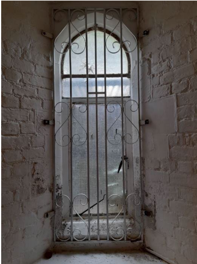
Crypt window, with holes
