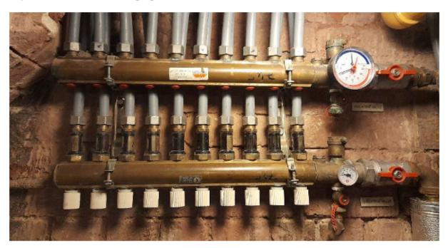
Black magnetic sludge can be seen in the sight glass flow meters of the underfloor heating manifold.
