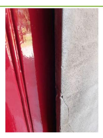
This image shows the door fully open with its outer edge in the curved recess. The thin stone edge which continues over the door is a good location for a draught seal strip. An alternative would be to install a strip fixed to the door itself to locate against this stone edge when closed.
