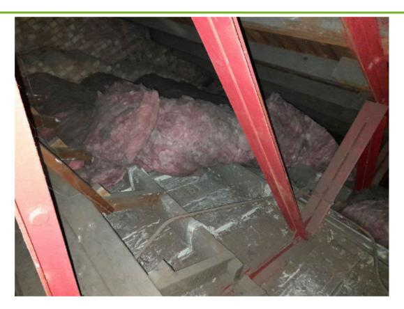
In all cases where there is 100mm or less of insulation within accessible roof spaces it is recommended that insulation be added to prevent heat loss and create a more comfortable environment for the occupants of the building.
