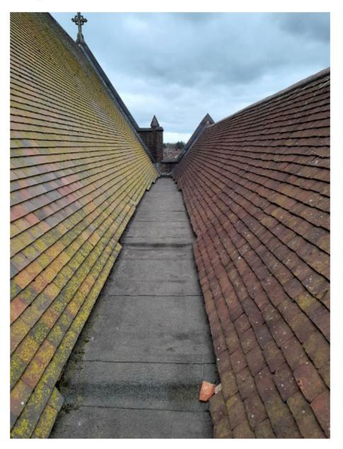
The roofs offer a useful area of around  $300\text{m}^2$ , considering two areas of 30m length x 5m drop over the nave and south aisle roofs. Installers should be asked if the more shaded aspect of the north aisle roof offers a potential site for the most recent and efficient type of panel.
