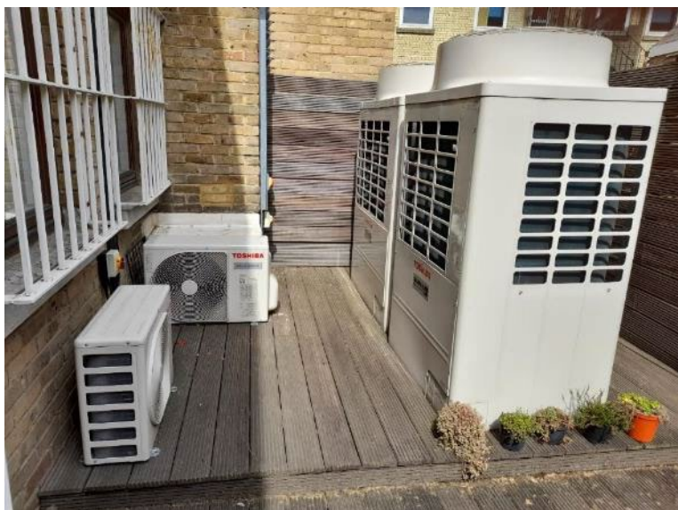
Examples of external units for AASHP comprising of three smaller 3kW units (output 10kW each) and two larger 10kW units (output 37kW each).
