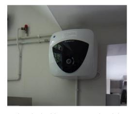
FST77. They should be set up with times to match the times that the building is occupied and this will prevent the standing losses from the unit wasting energy during periods when the building is not occupied.
