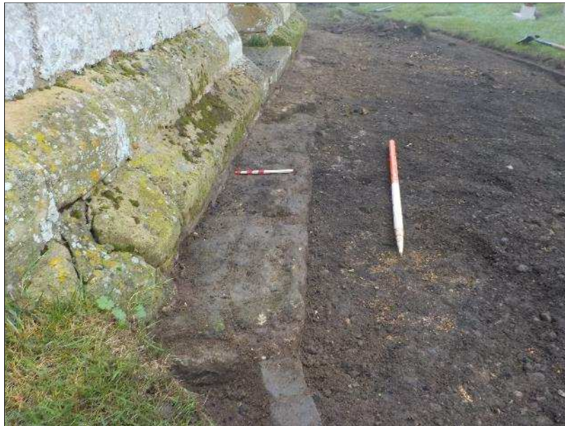
Plate 3: Foundation slab 103 and stepped footings of church tower, looking south. Scales 1m and 0.3m
