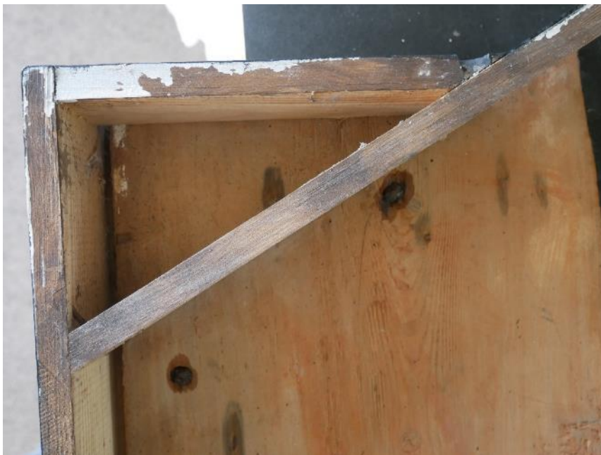
Fig 9 Note construction of added box frame.
