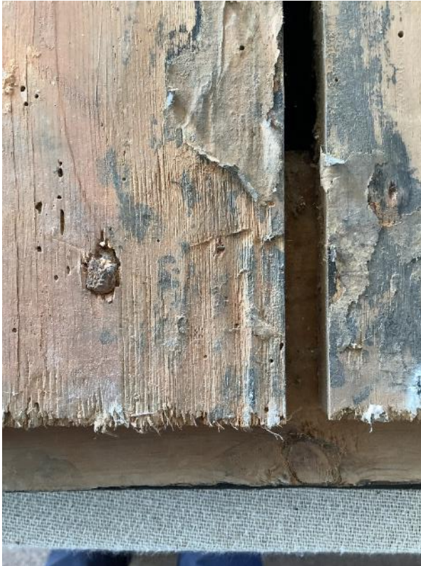
Fig 8 There is no additional frame at the bottom of the boards so allowing good air flow behind.
