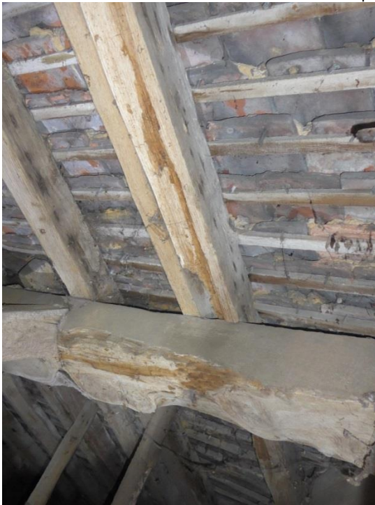
Tiles on north nave roof slope, as existing.
