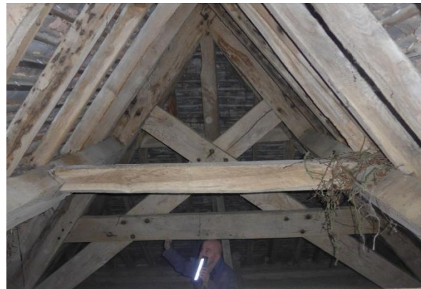
North chapel roof interior, as existing.
