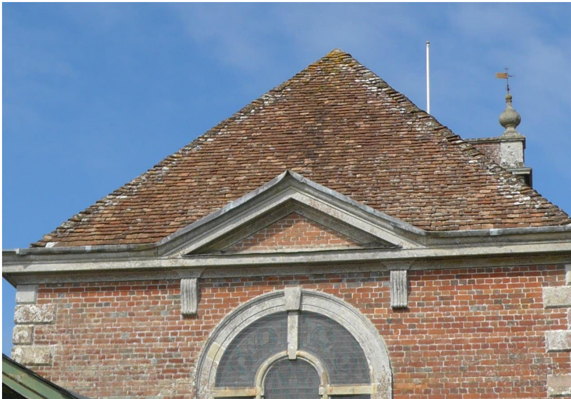
East facing hipped roof over Chancel
