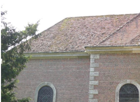
North Chancel Roof
