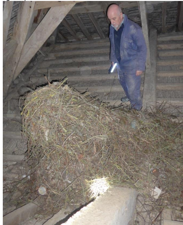
Nesting material for clearance in N chapel roof.
