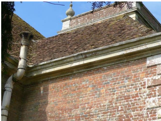
East side of North Chapel Roof
