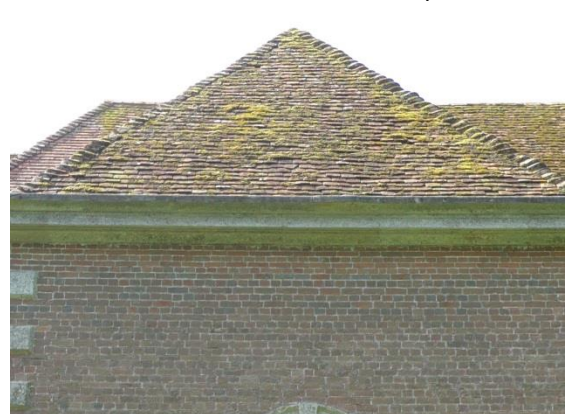
North facing hipped roof over North Chapel
