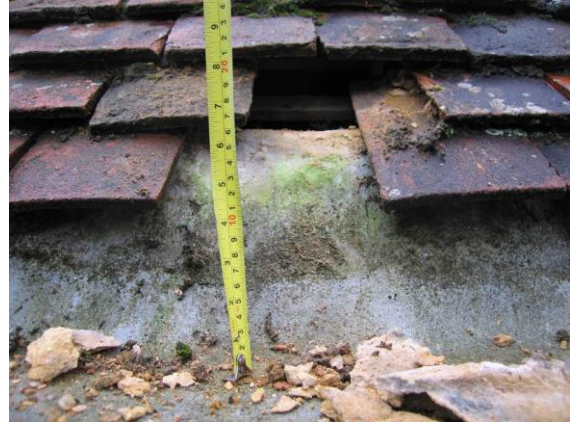
Typical section of existing cornice weathering, with top edge exposed
