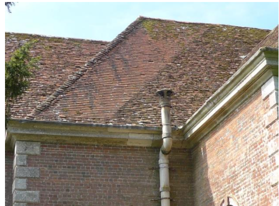
Eastern end of North Nave Roof Slope
