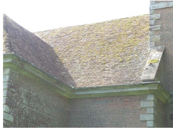
Western end of North Nave Roof Slope
