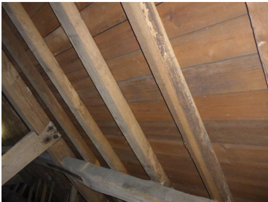
Chancel roof boarded and felted, as ex.g.
