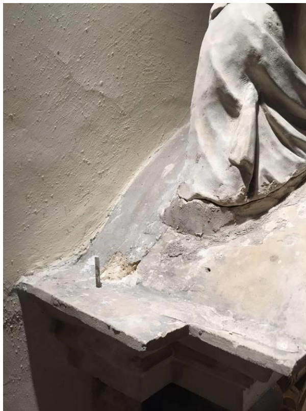
Fixing for west side flame finial
