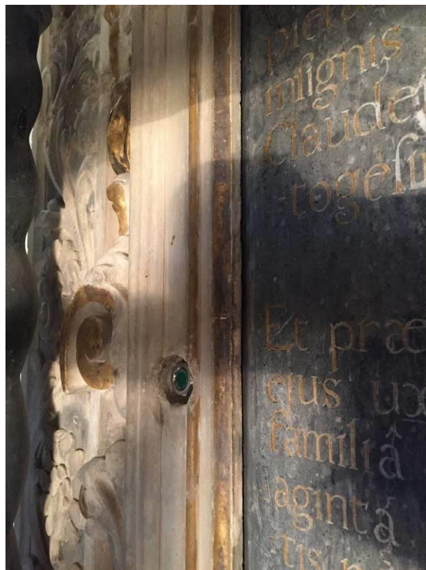
Fixing to west side of inscription tablet before and after replacing with stainless
