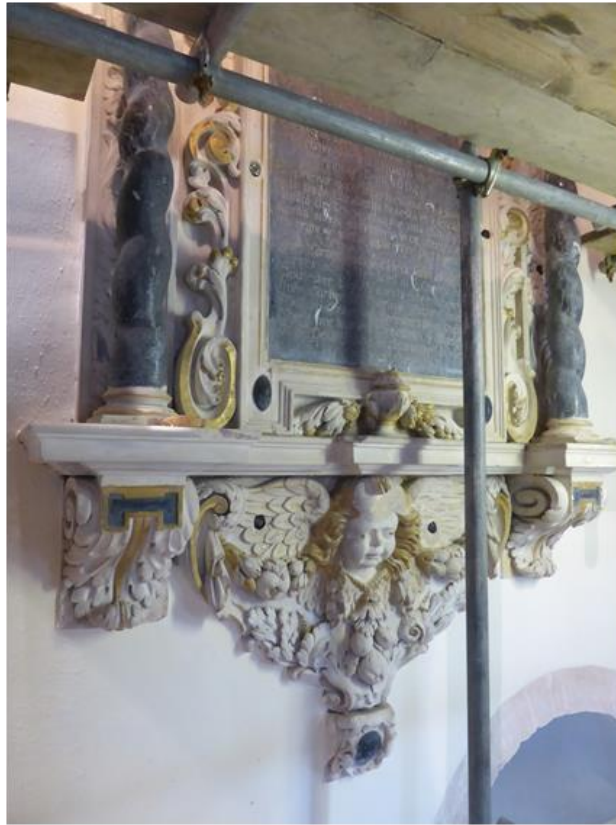
Lower half of monument with exposed ferrous fixings treated
