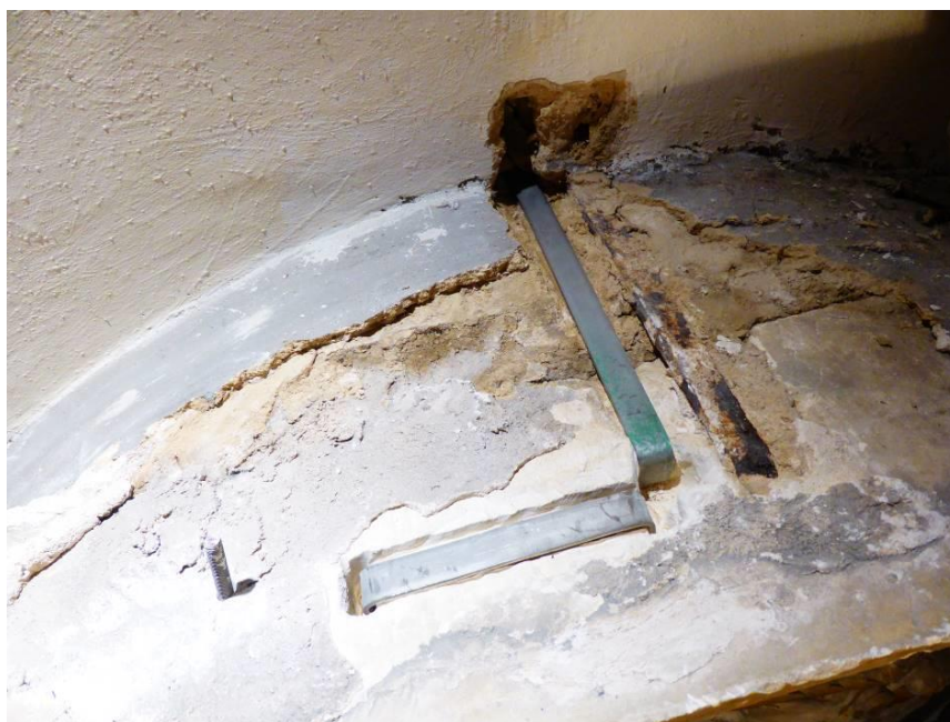
During fitting of replacement cramps and locating dowel for west cherub
