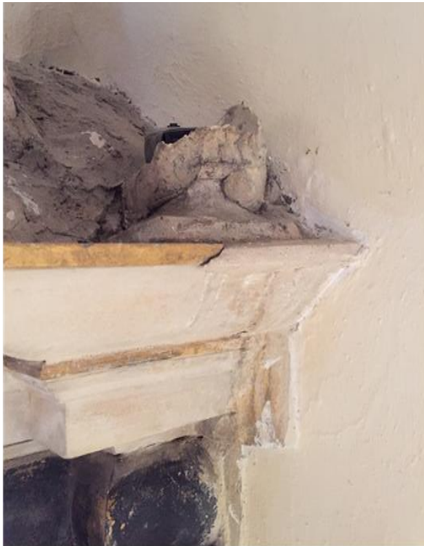
East side finial socle before treatment
