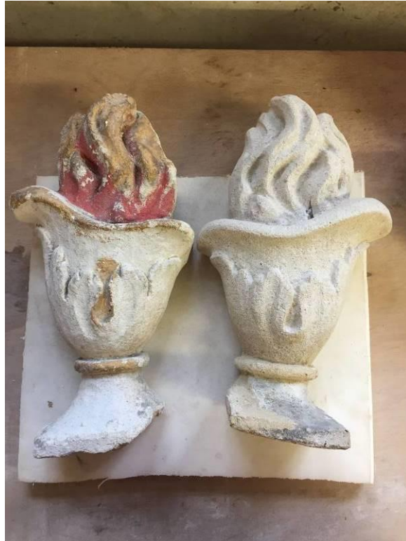
West side urn and newly carved east side urn on original socle, prior to retouching to match
