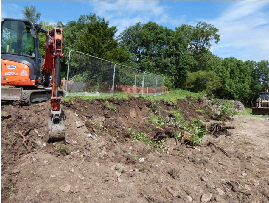
Pl. 1: View of site from S during removal of former boundary wall
