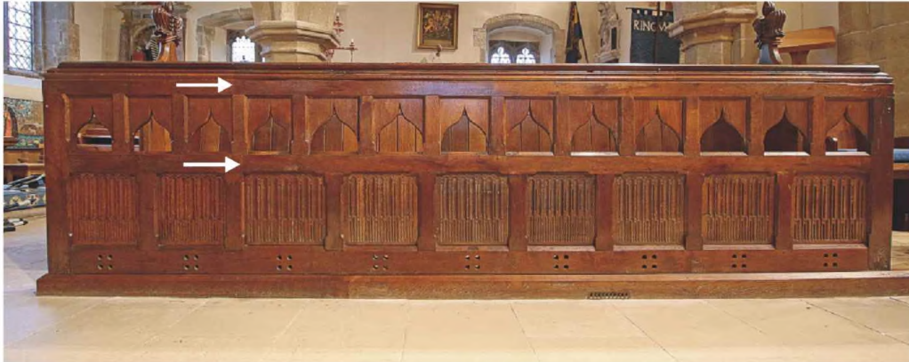
5. Front to south stalls. Most of this front is ancient except the left hand two panels, arrows show joints in rails.
