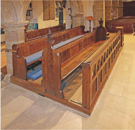
4. Oblique view of south stalls
