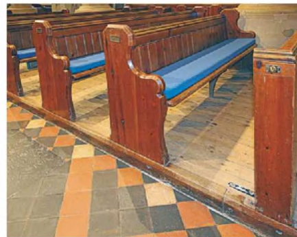
22. Typical pews as seen in the nave
