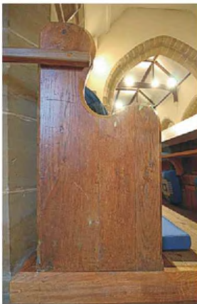
6. East end to south stalls; note end made from 3 planks of unequal width.
