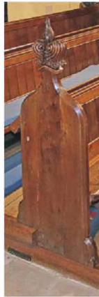
7. Front stall end also made from 3 planks
