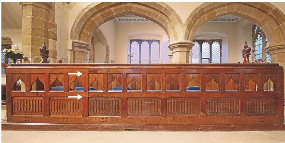
15. Front to north stalls. Most of this front is ancient except the left hand two panels, arrows show joints in rails.
