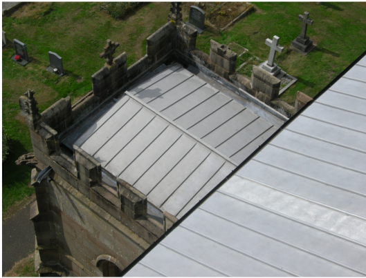
Roof and Parapet
