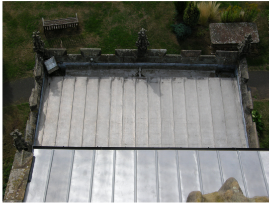
Roof and Parapet
