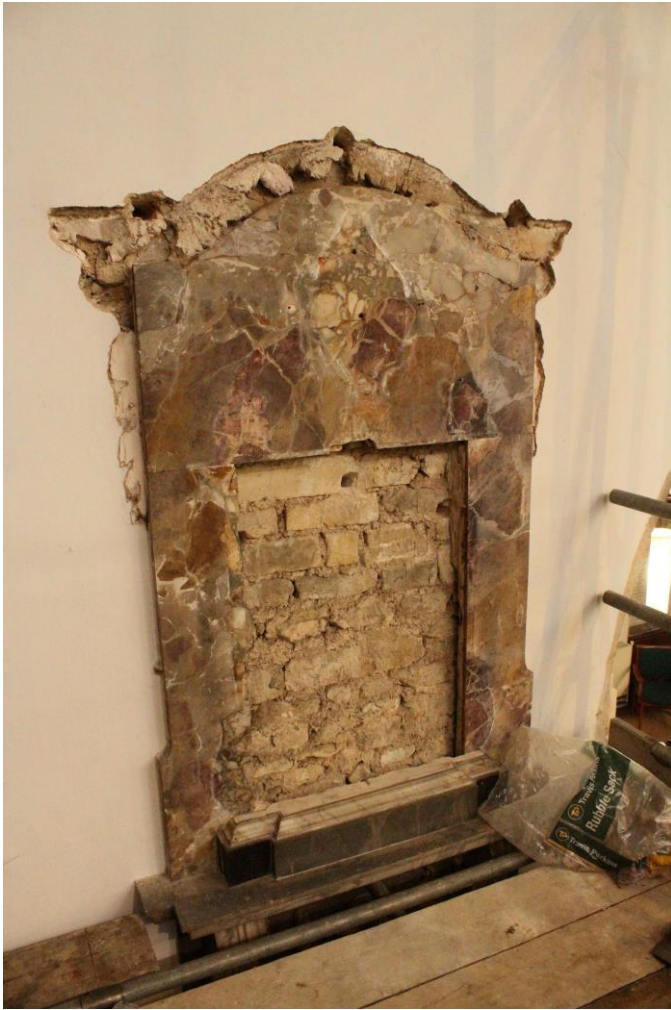
Work in progress, clockwise from left: the monument at fullest extent of dismantling; mixing and laying plaster for refixing; fixing a bracket into place; cleaning with cotton wool swabs
