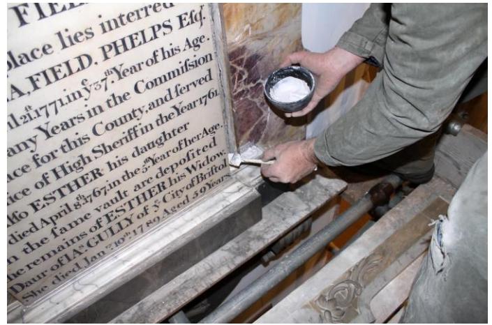
Work in progress, clockwise from left: the monument at fullest extent of dismantling; mixing and laying plaster for refixing; fixing a bracket into place; cleaning with cotton wool swabs
