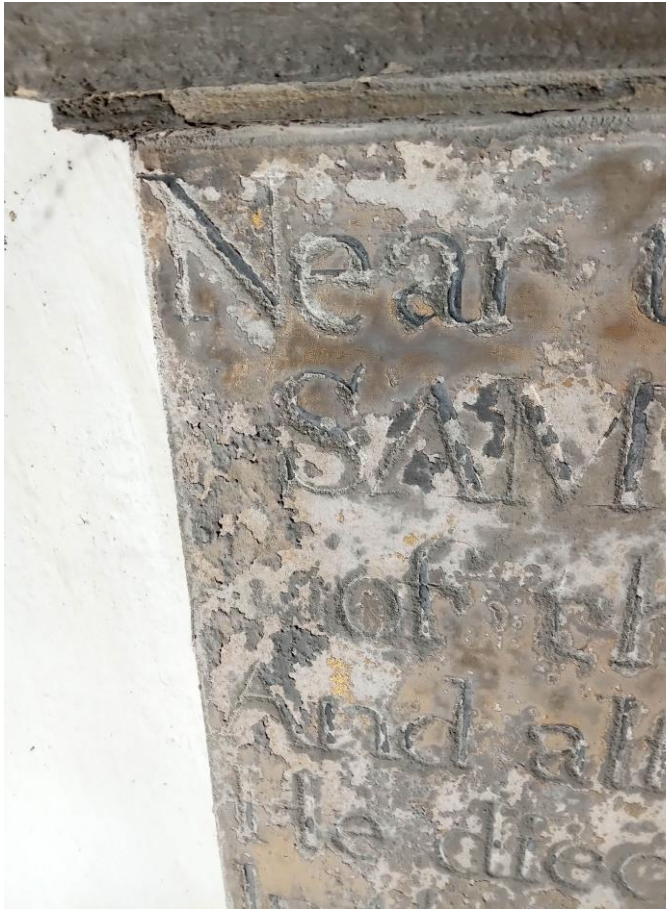
Above: flaking paint in the letters of the inscription; above right: cleaning in progress; below partially dismantled, note iron fixing and gilding emerging from under overpaint
