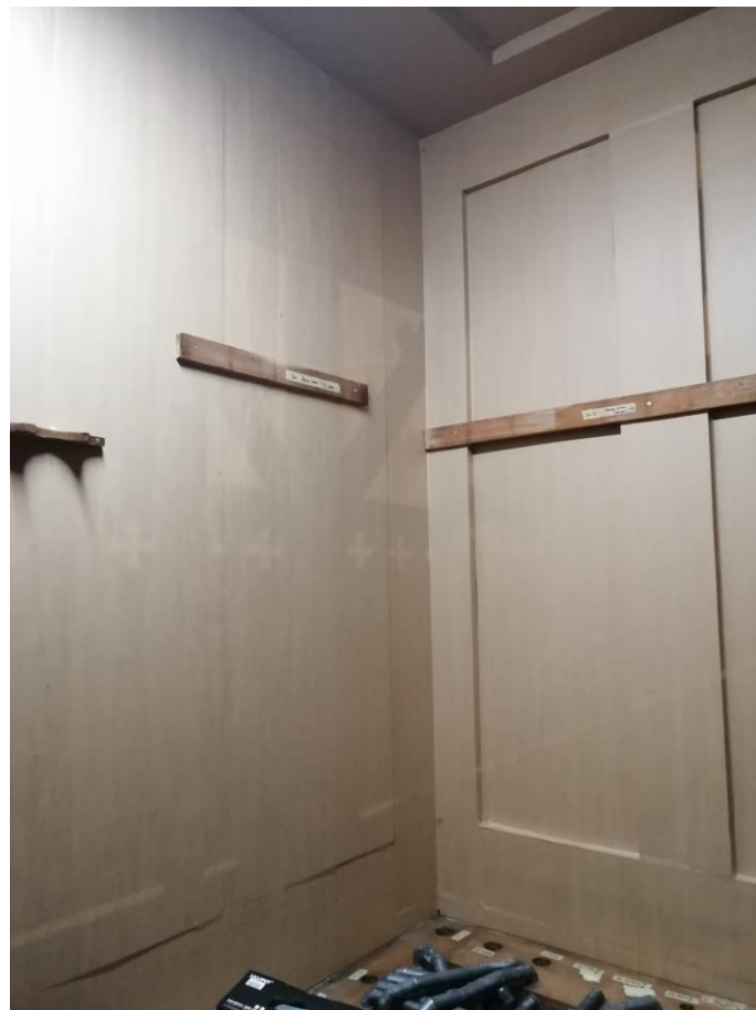
Re-lined box interior
