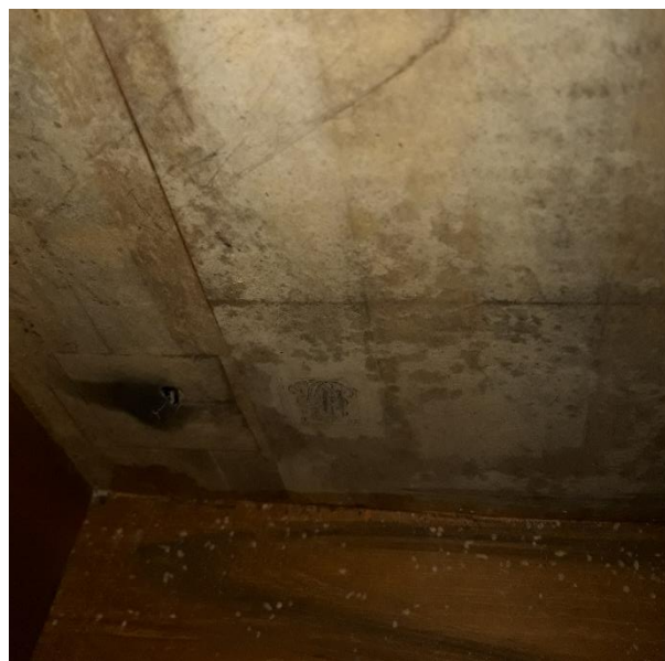
Grid covering at St John the Baptist Church, Healaugh formed of paper pieces
