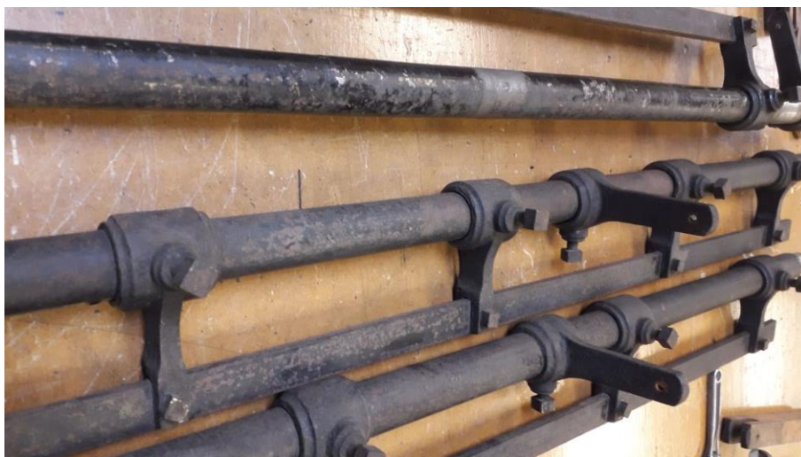
State of metalwork before restoration
