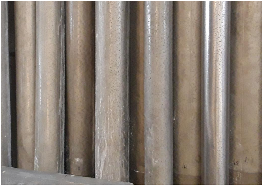
Façade pipes as removed, with one (second from right) restored to original condition
