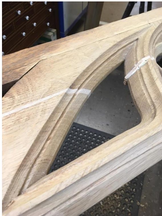
Repairing splits by piecing in new timber: there were countless such repairs to be made
