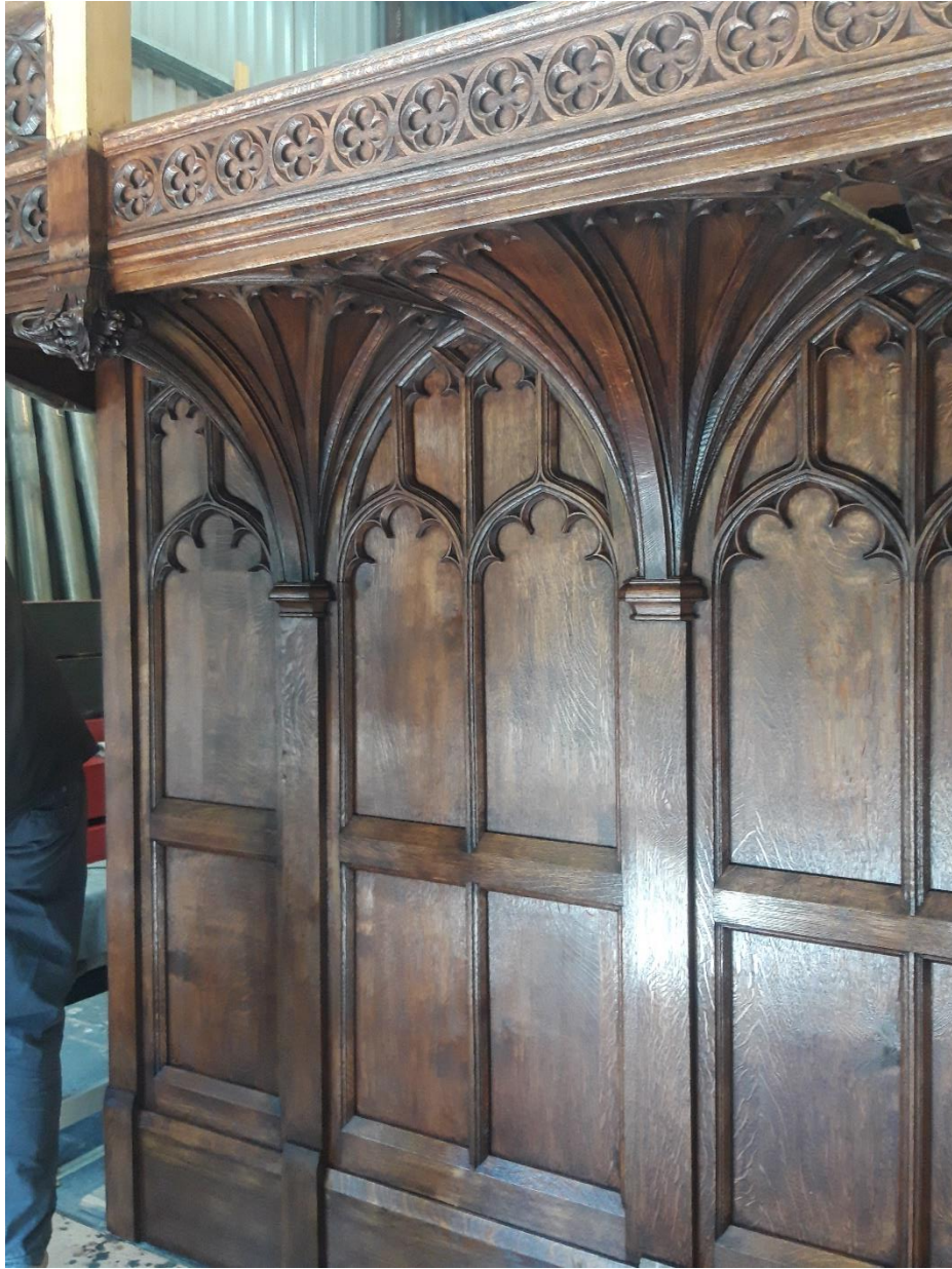
Timber fan vaulting after stripping, repair, staining and polishing
