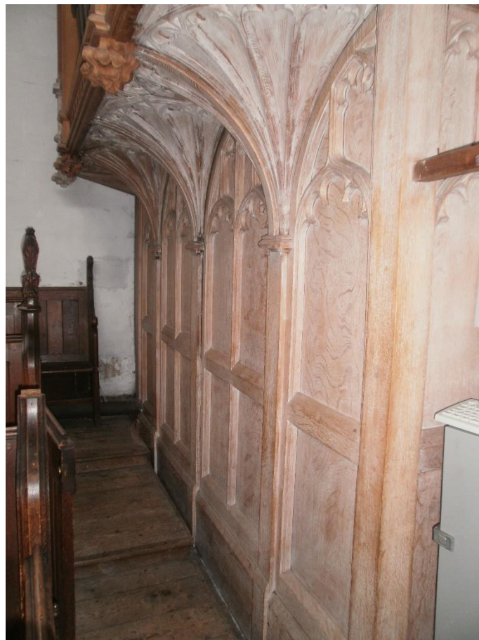
Timber fan vaulting before restoration
