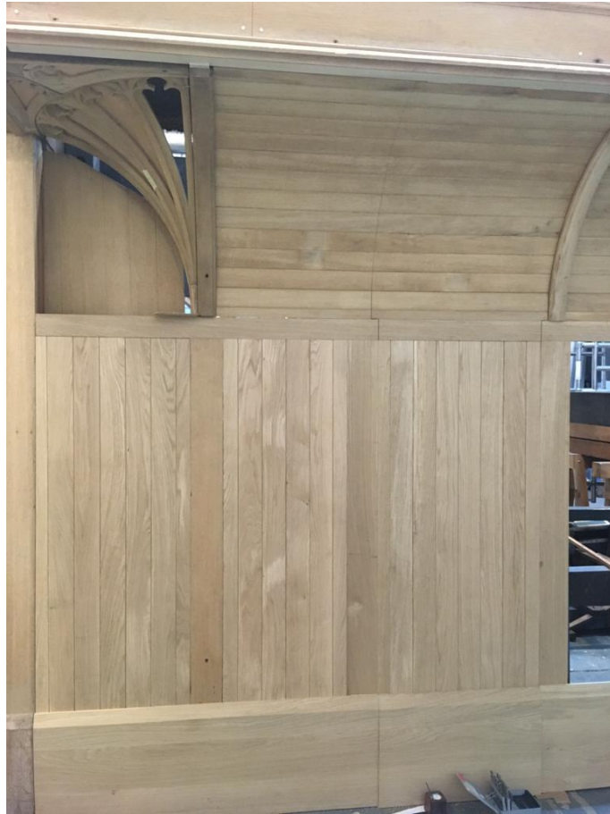
The new casework on the right-hand side of the instrument, before staining and polishing
