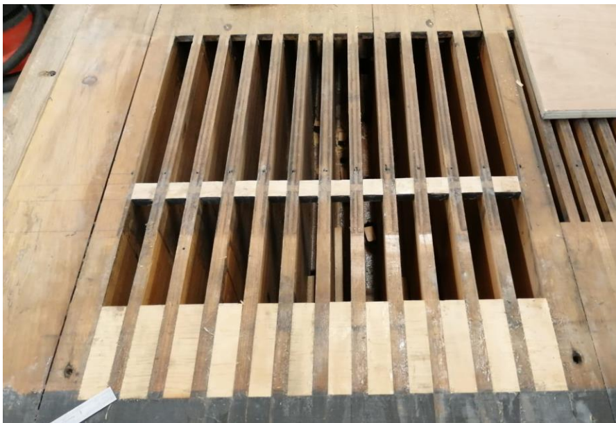
New infills in Swell Organ soundboard
