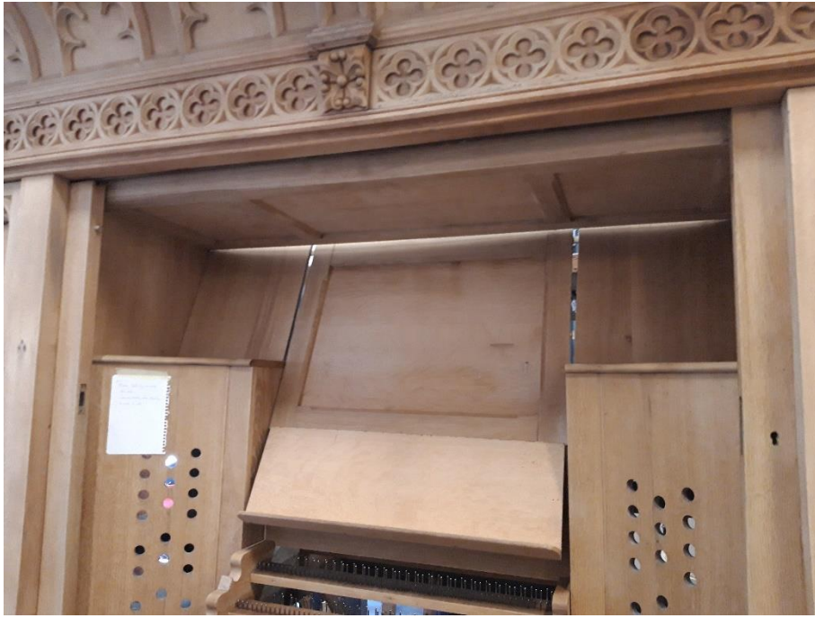
Stripped console during restoration
