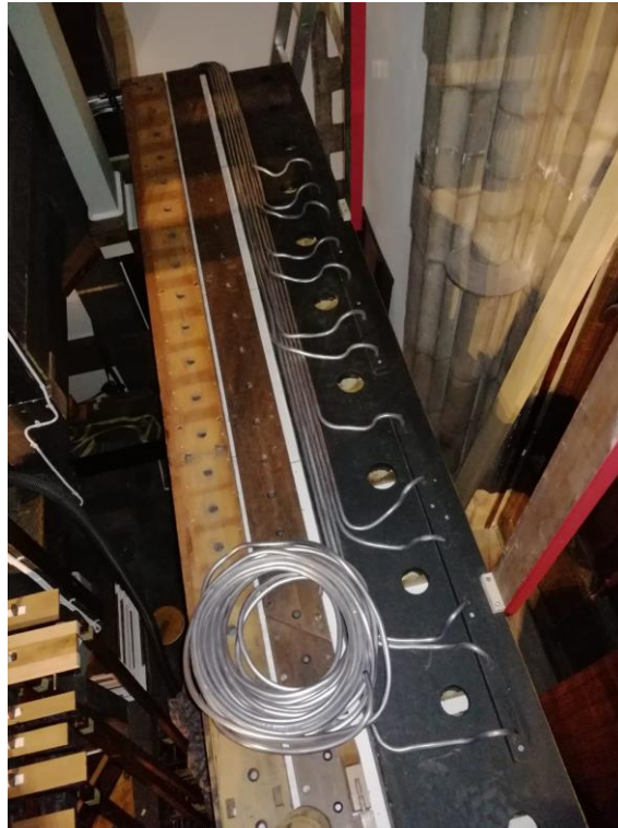
Running new lead tubing
