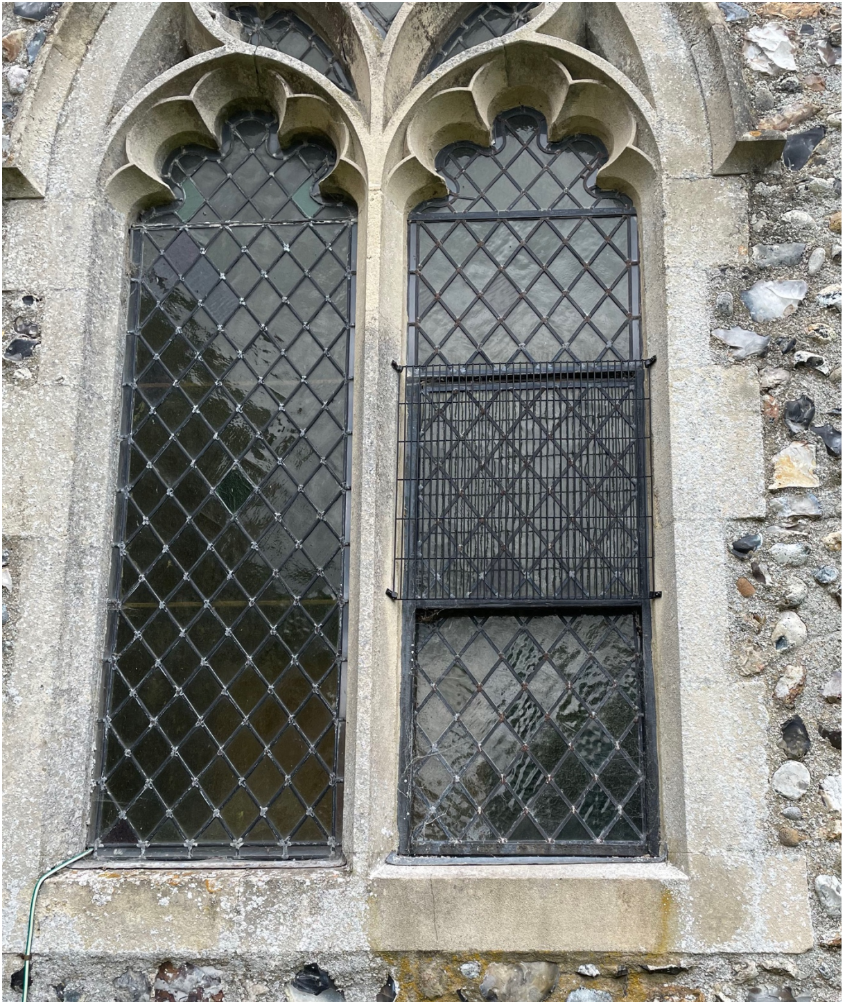
Figure 2: East Facing Window North Aisle
