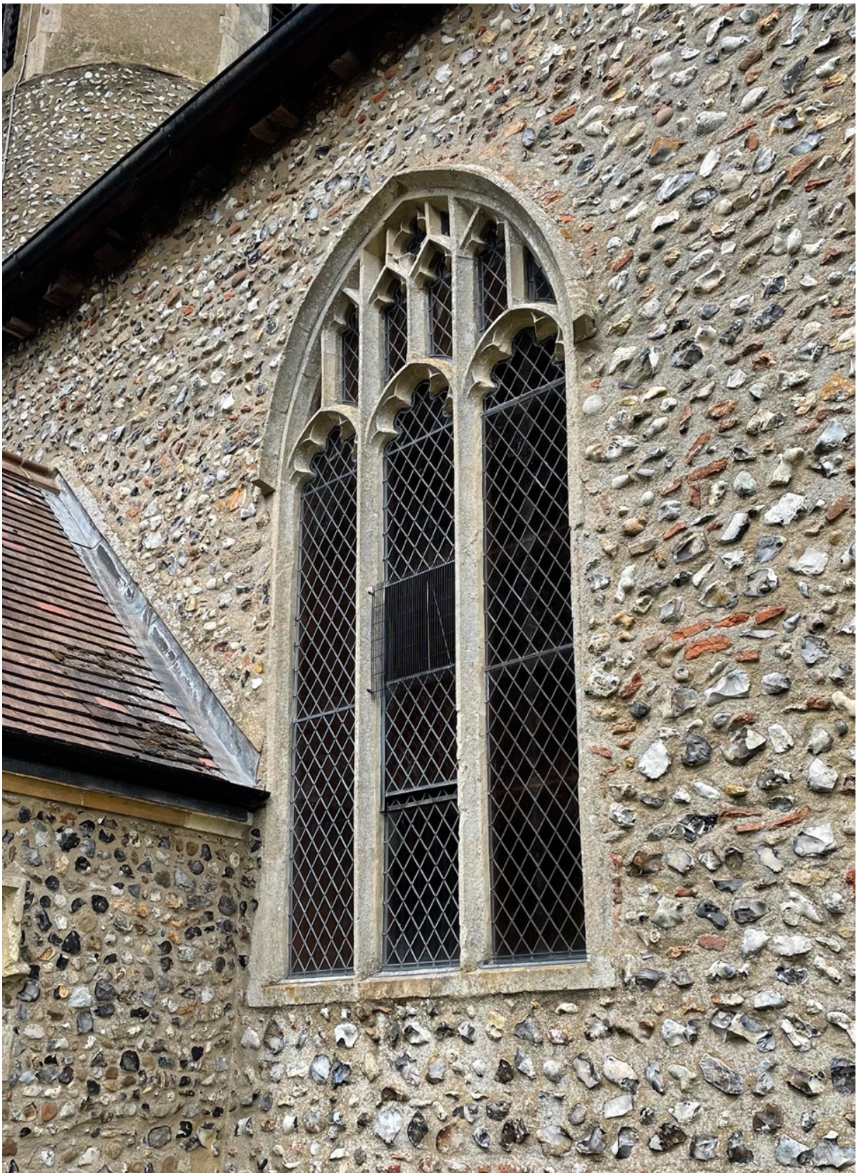
Figure 3 - Western South Facing Window in Nave
