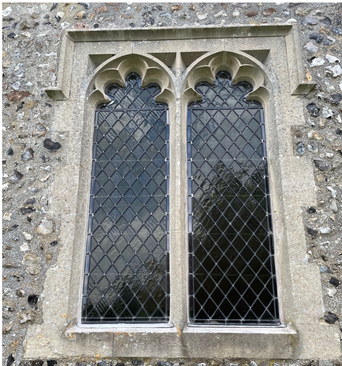
Figure 1 - North Window of North Aisle
