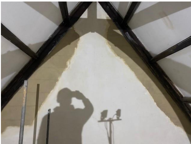
Plaster work in progress:
