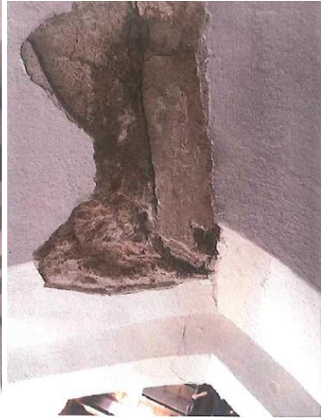
Wall plaster - various patches of failing plaster:
