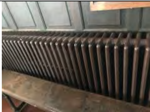
No suspect ACMs behind
