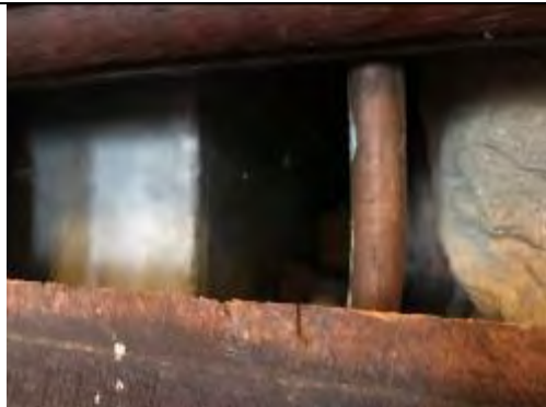
Stone and timber behind. No suspect ACMs
