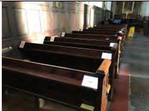
Pews to be removed
