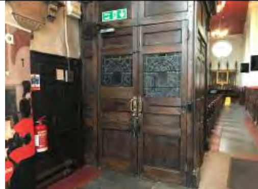
Timber doors to Porch
