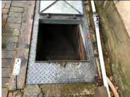
Access to Boiler Room
