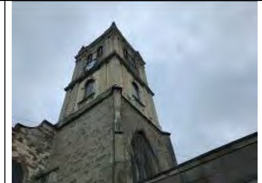
Tower no access above Ground Floor
