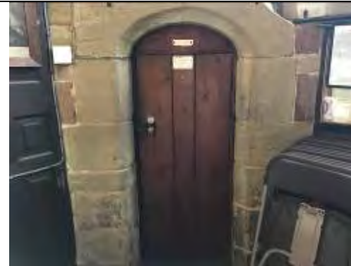
No Access to Tower. Not included in scope of works
