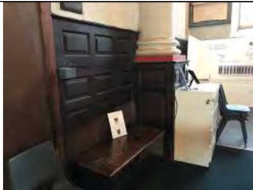
Timber panels to walls and solid column
