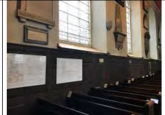
Timber panels to walls
