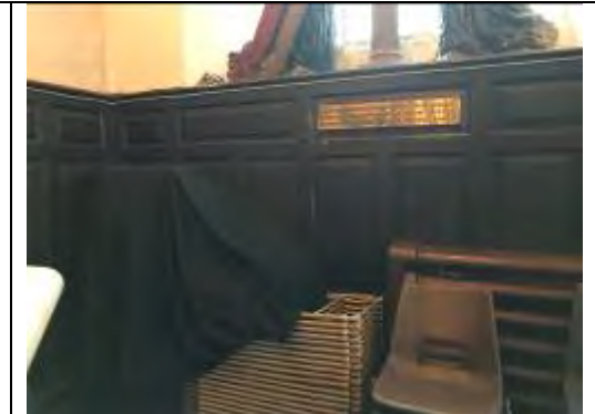
Timber panels to walls
