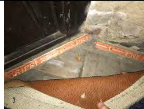
Parquet flooring below
