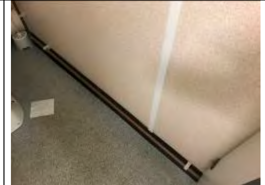
Modern non ACM flooring and skirting
