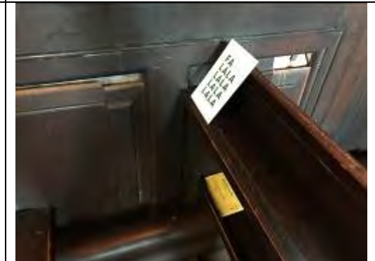
Timber panels to walls
