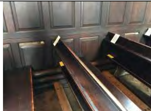
Timber panels to walls
