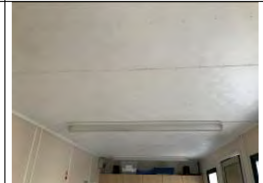
Non ACM boards to ceiling
