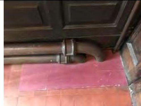
Cast pipes extending down through floor
