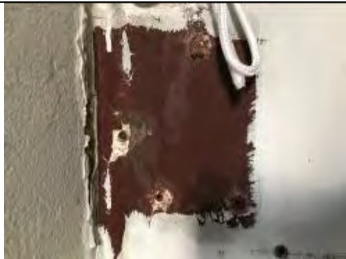
Plaster on solid walls
