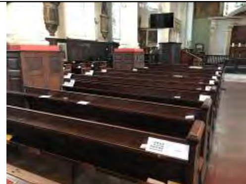
Pews to be removed
