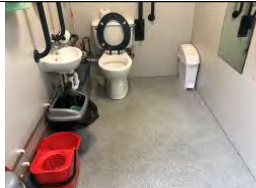
Modern non ACM toilet suite and flooring
