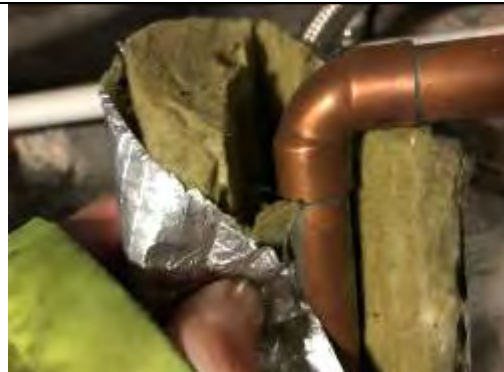
No debris to pipes
