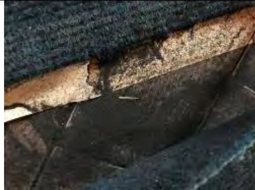
Parquet flooring below
