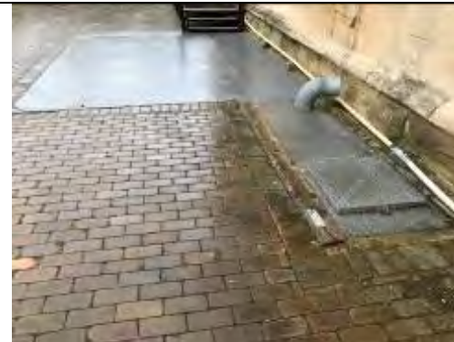
Access to Boiler Room
