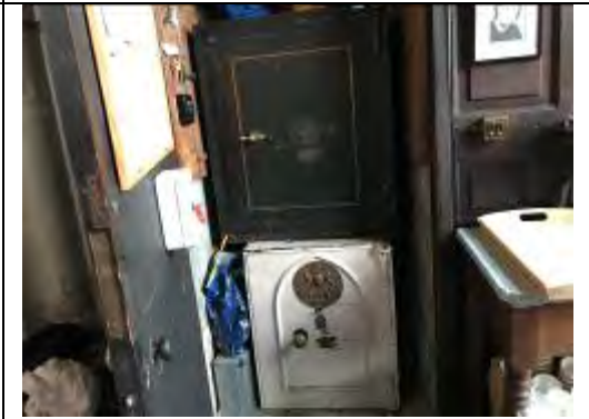
Presumed asbestos insulation board laminate to safes Crocidolite
