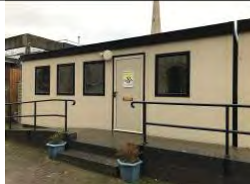
Kitchen within Portacabin
