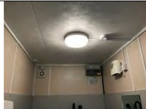
Modern non ACM lining to walls and ceiling
