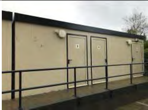
Toilets within Portacabin
