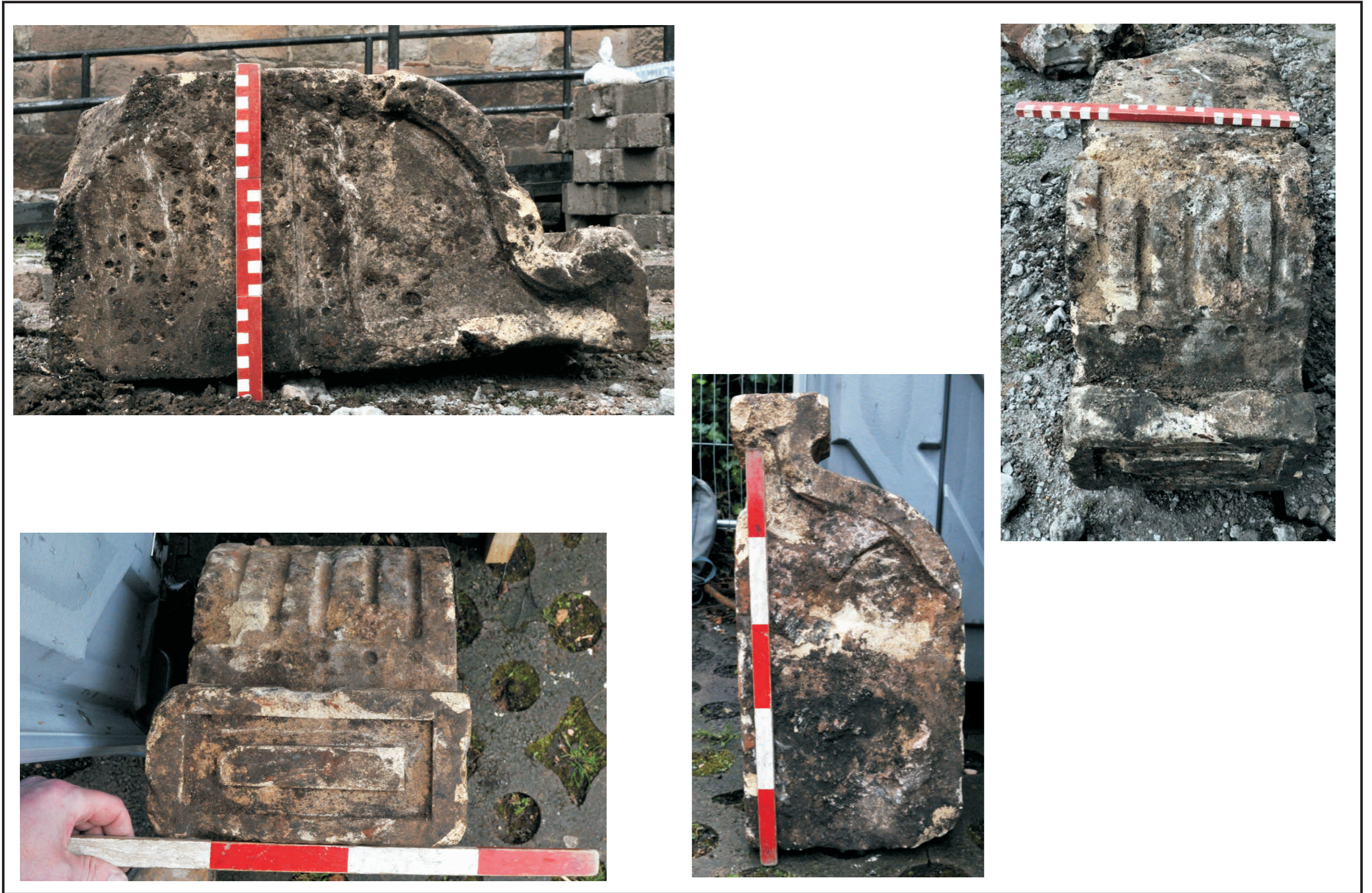
Figure 9: Substantial limestone corbel recovered from foundations of former vestry. Not retained (reburied on site) Approx dimensions 280x230x560mm.
