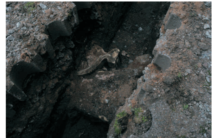
Corbel re-used in foundation
