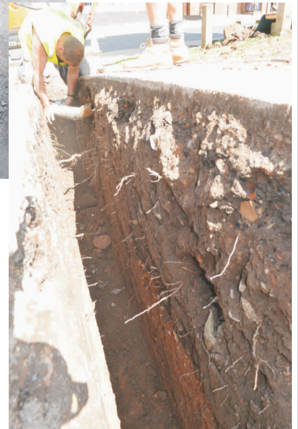
Same section of trench part excavated
