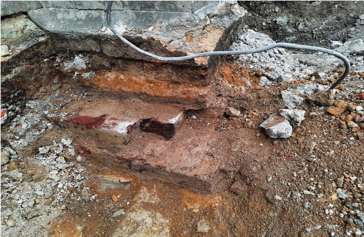
31) Under South Aisle SW buttress has had a number of bricks underpinning it. A brick size noted as wider than 4" and dating of the underpinning could be anything from the late C17th to late C18th
