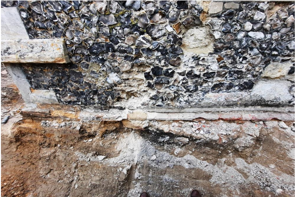
33) Small flint fall. Random foundation stones and bricks along this East end of the South Aisle
