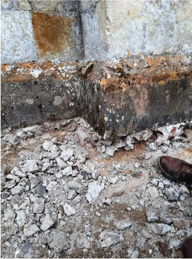
40) The foundation below the NE corner of the North aisle was again underpinned – this time in reinforced concrete
