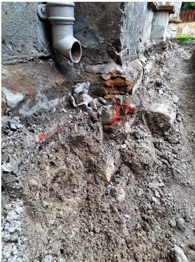
33) Small flint fall. Random foundation stones and bricks along this East end of the South Aisle
