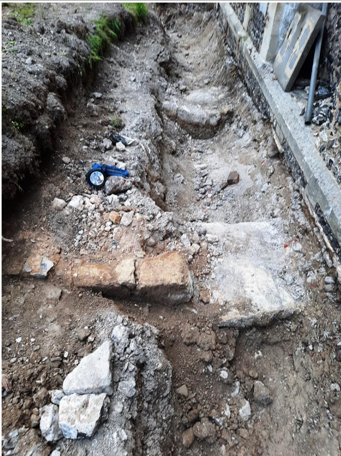
41) North wall had little supporting foundation of the applied flintwork –some has fallen away
