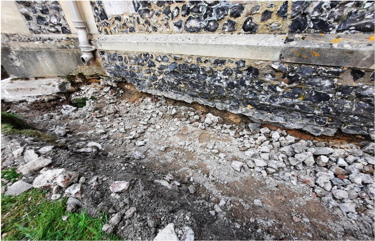
41) North wall had little supporting foundation of the applied flintwork –some has fallen away
