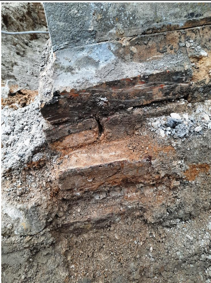
31) Under South Aisle SW buttress has had a number of bricks underpinning it. A brick size noted as wider than 4" and dating of the underpinning could be anything from the late C17th to late C18th
