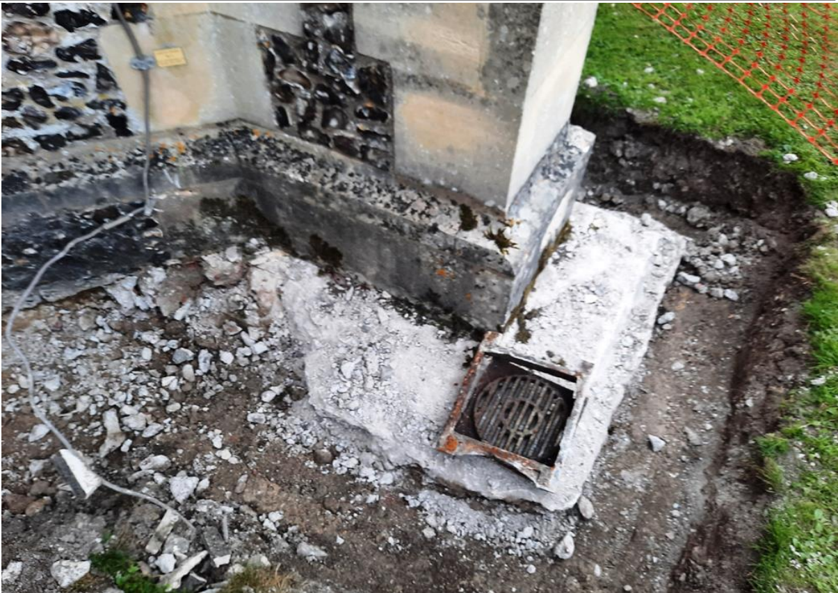
40) The foundation below the NE corner of the North aisle was again underpinned – this time in reinforced concrete
