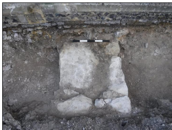
Plate 6: West side of N-S foundation of porch [3] ( Scale = 500mm )
