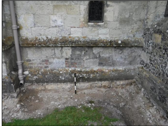
Plate 13: Detail of wall and footings at NW end of chancel.
