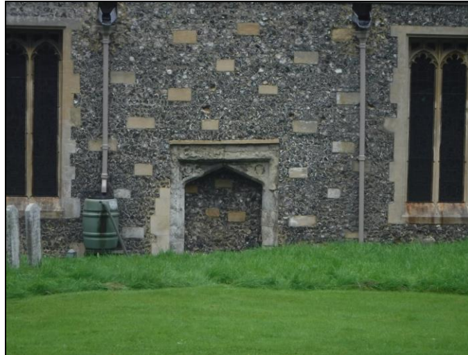
Plate 1: Detail of blocked doorway of former porch
