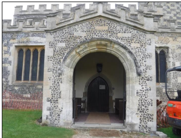
Plate 12: Entrance to existing porch on N side of church looking south
