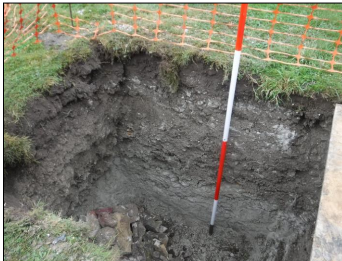
Plate 14: Detail of soakaway at the SE corner of the church view ESE
