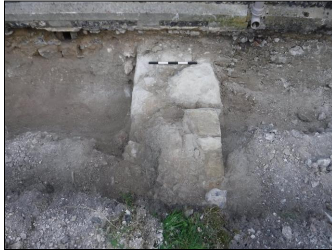
Plate 7: East side of N-S foundation of porch [4] ( Scale = 500mm )
