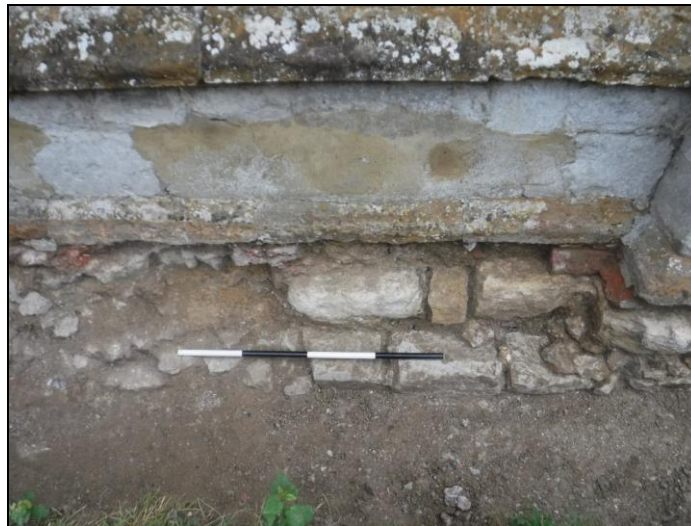
Plate 11: Footings of chancel on its south side ( Scale = 1m )
