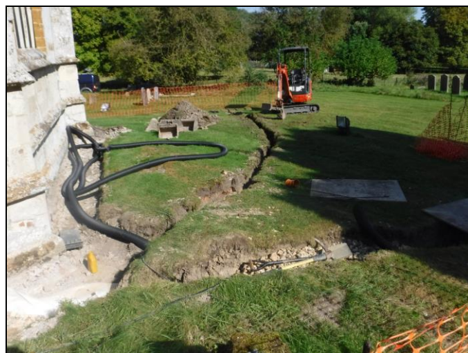
Plate 15: Drainage run on the east end of the church view west
