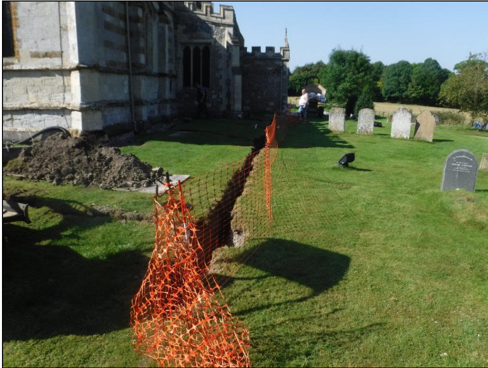
Plate 16: E-W drainage run looking west on north side of the church
