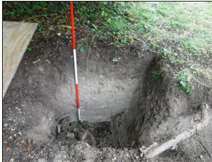
Plate 2: Detail of soakaway on SW side of church view N
