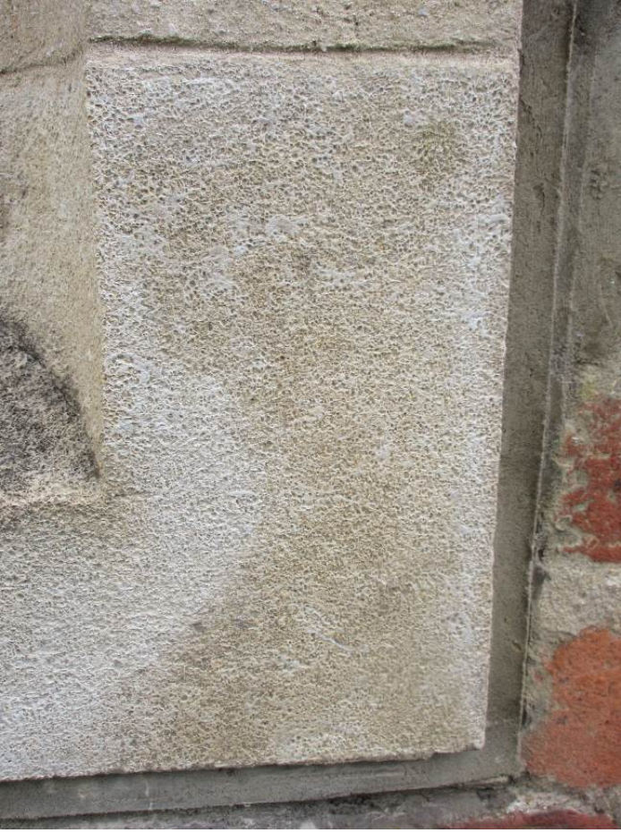
Plate 4a Stone window sill in Clipsham stone
