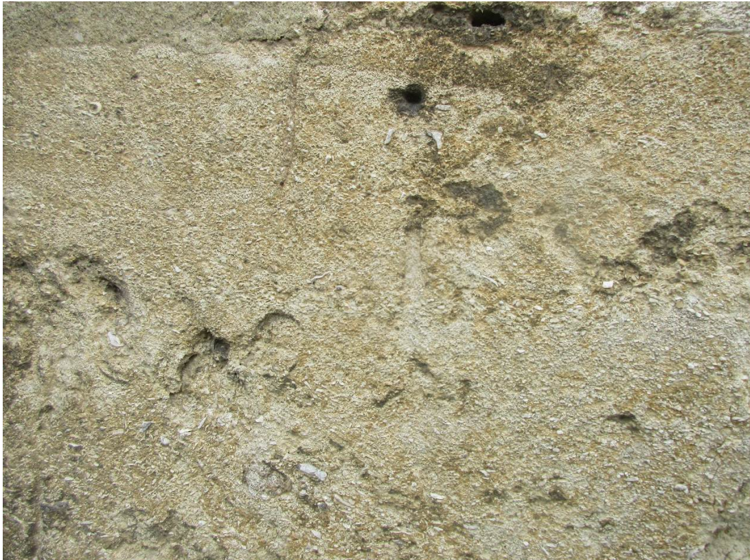
Plate 3a Close up of Headington stone in the jamb of the east window
