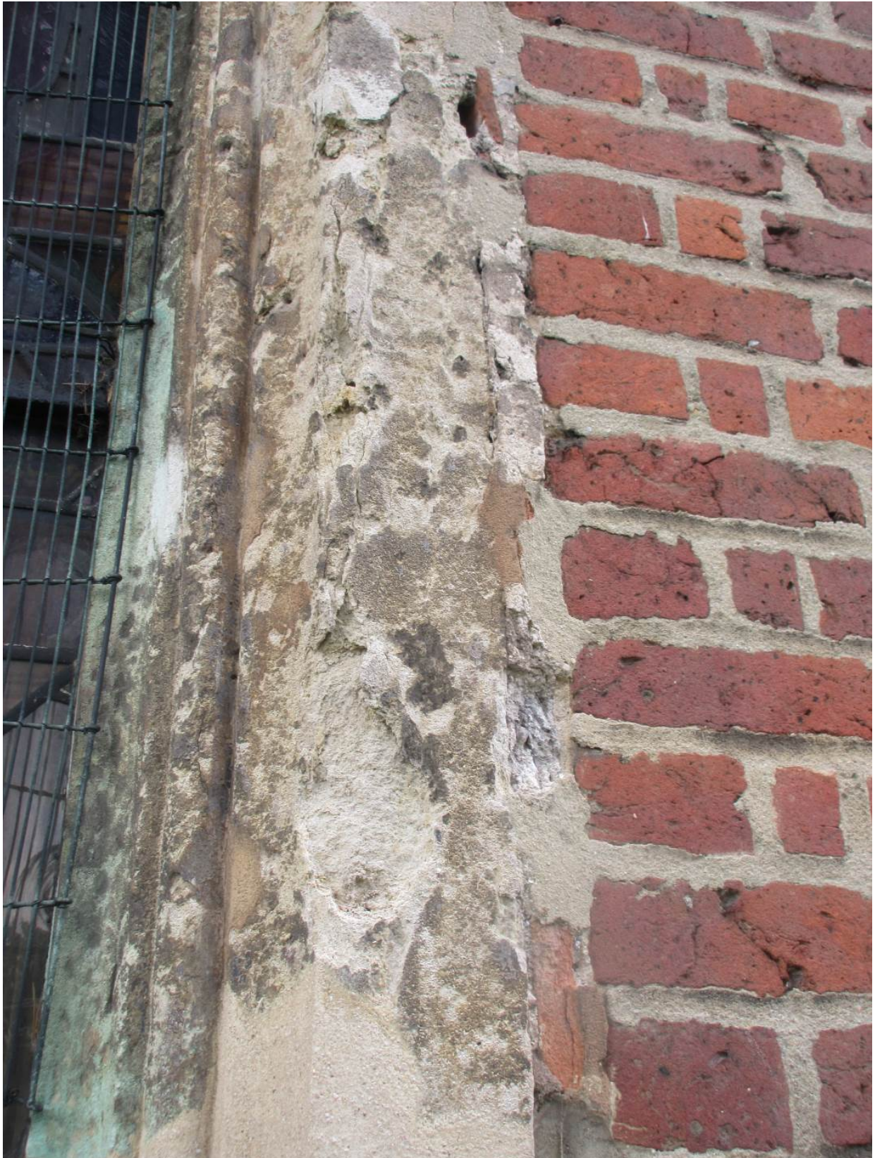
Plate 2 Blistering of Headington stone in the jamb of the east window
