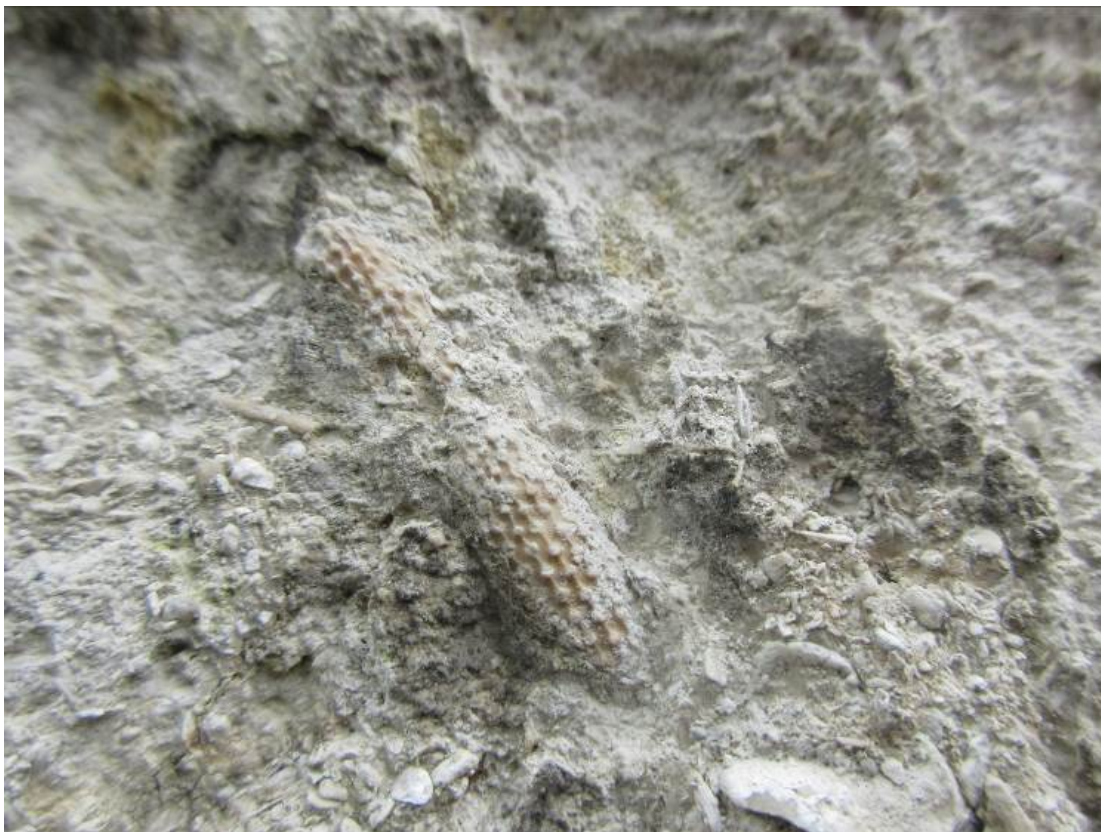
Plate 3b Close up of Crinoid Plegiocidaris florigemma in north-east quoin of St Lawrence Church, typical of Headington stone (Upper Jurassic) Oxfordshire
